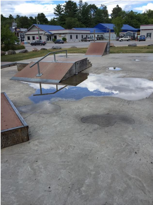
**Figure 2 - As we can see our current skate park lacks proper drainage systems, this is due to the soil below the concrete unfortunately. Everyone here can agree, this needs to be addressed. Photo by Trevor Kelly**
