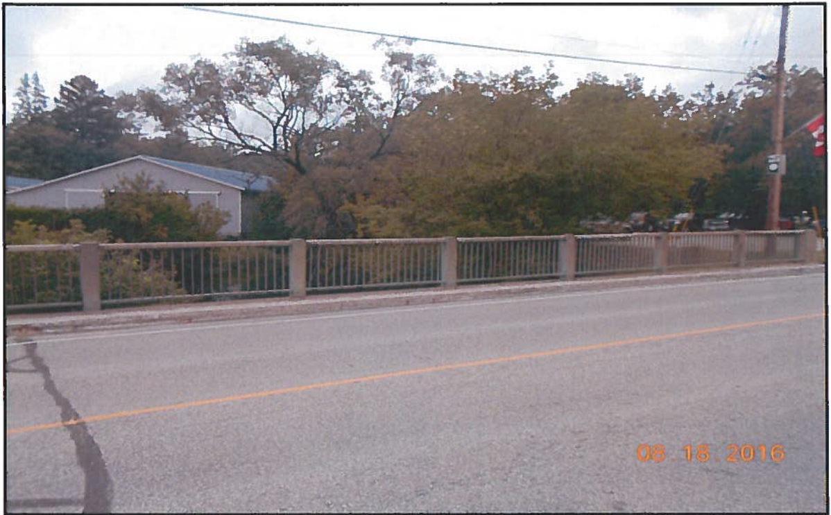
Photo 5 : General View of Handrail System- Looking East
