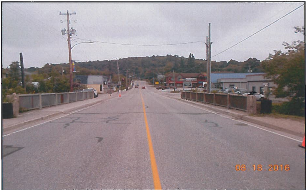
Photo 2 : General Arrangement - Looking North
