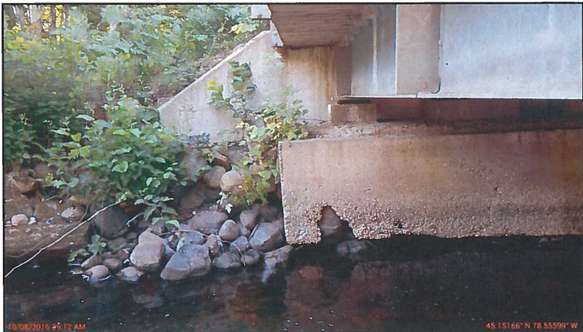
Photo 6 : General Arrangement – Southeast Embankment at Abutment
