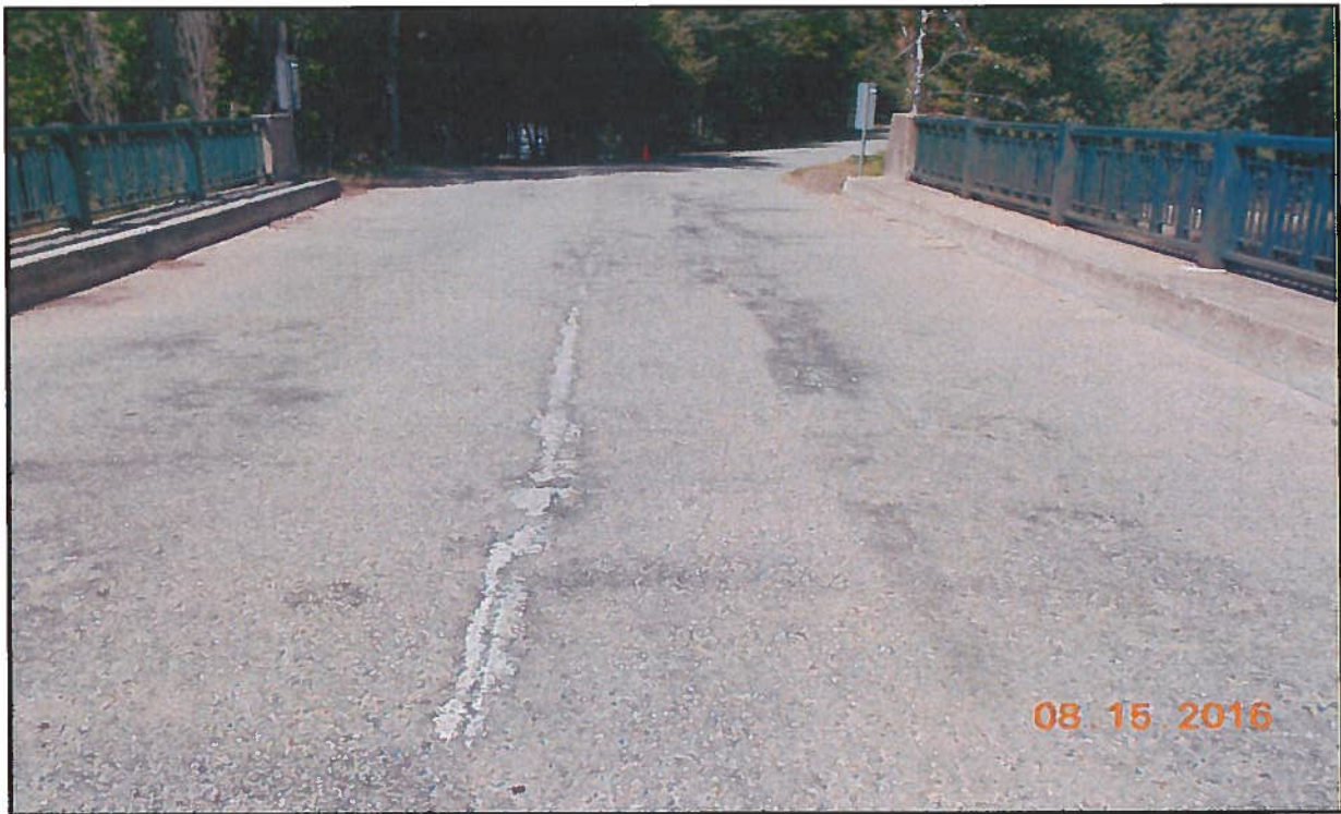
Photo 5 : Deck Wearing Surface – Looking West
