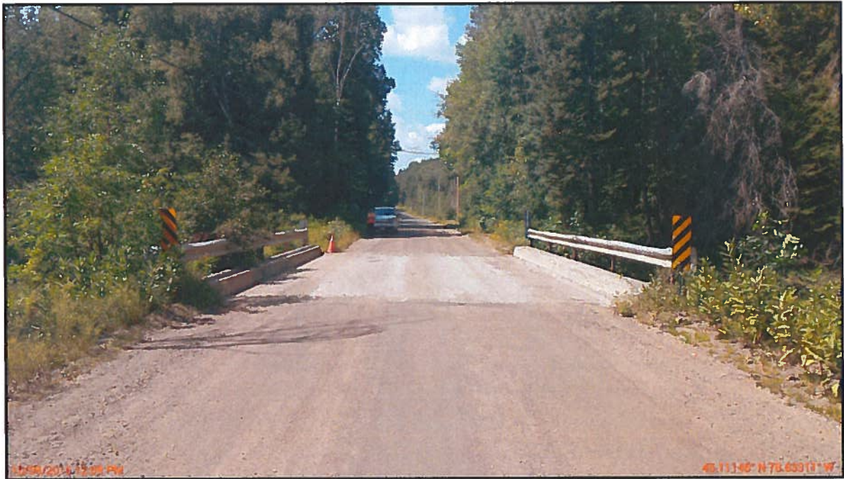
Photo 2 : General Arrangement – Looking West
