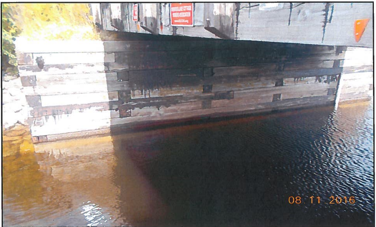
Photo 6: General View – West Abutment
