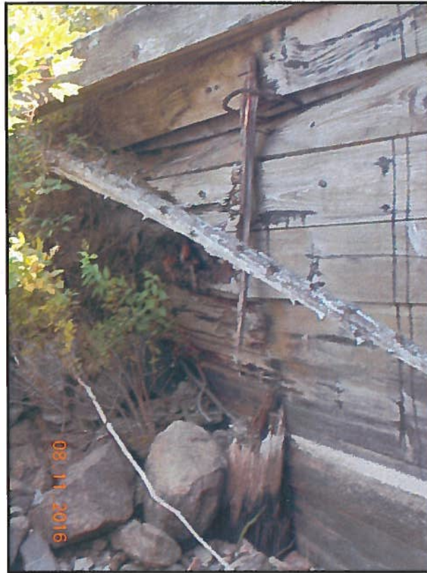
Photo 9: Northeast Abutment Wing Wall – Looking Southwest
