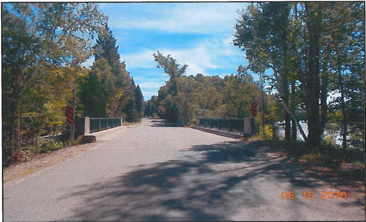
Photo 2 : General Arrangement - Looking East
