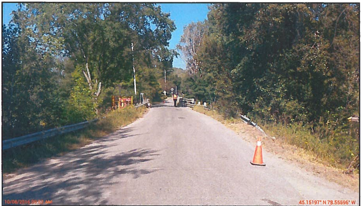
Photo 2 : General Arrangement – Looking West
