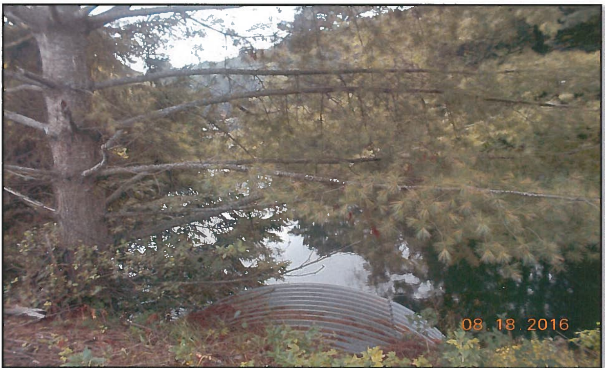
Photo 4 : General Downstream View – Looking West
