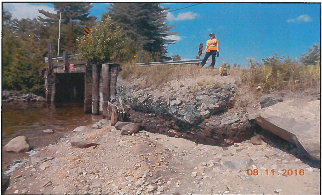
Photo 4: General Arrangement – Southeast Embankment
