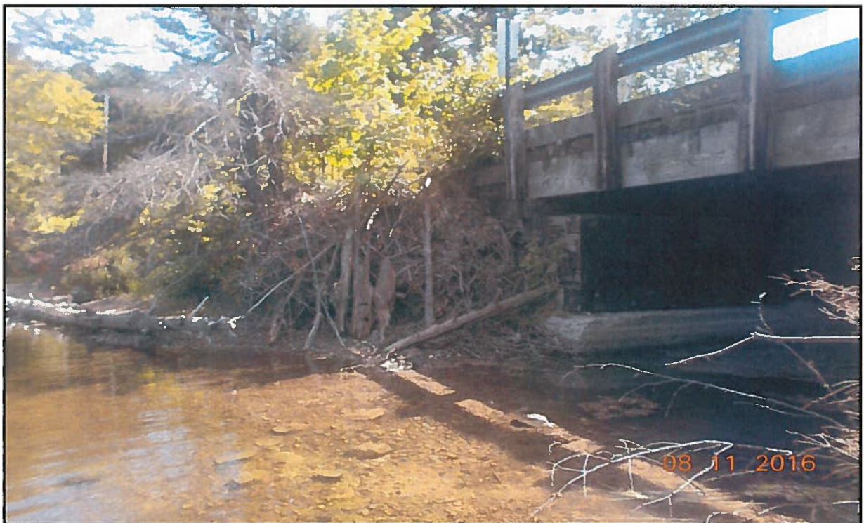
Photo 4 : Northwest Embankment – Looking North
