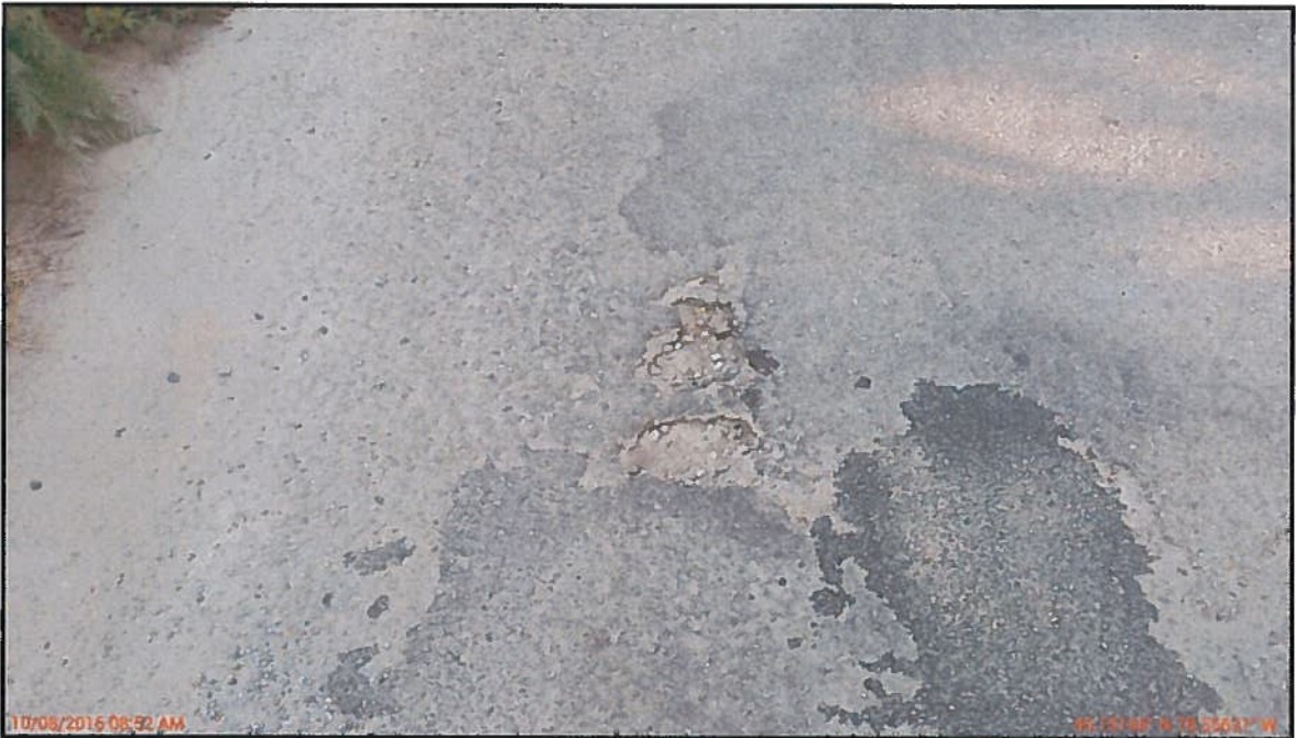
Photo 12 : South Approach Wearing Surface – Looking South
