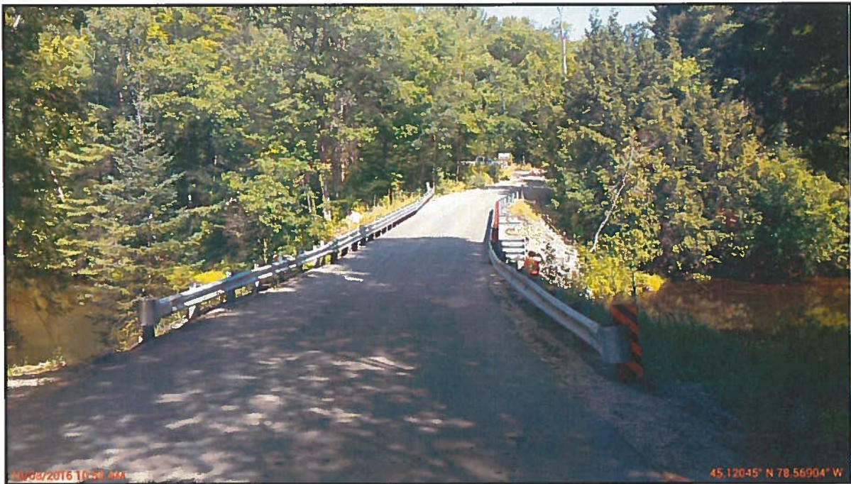
Photo 1 : General Arrangement - Looking North
