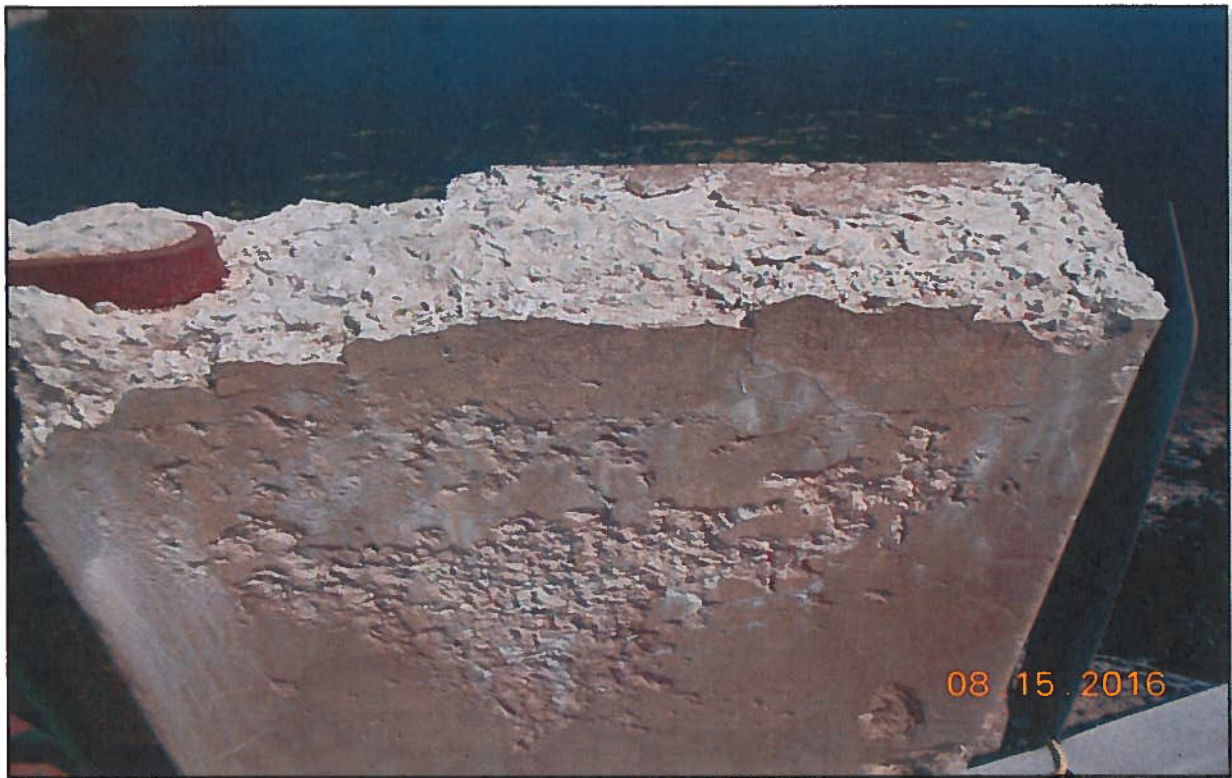
Photo 6 : Typical Concrete End Post of Handrail System - Southeast Quadrant
