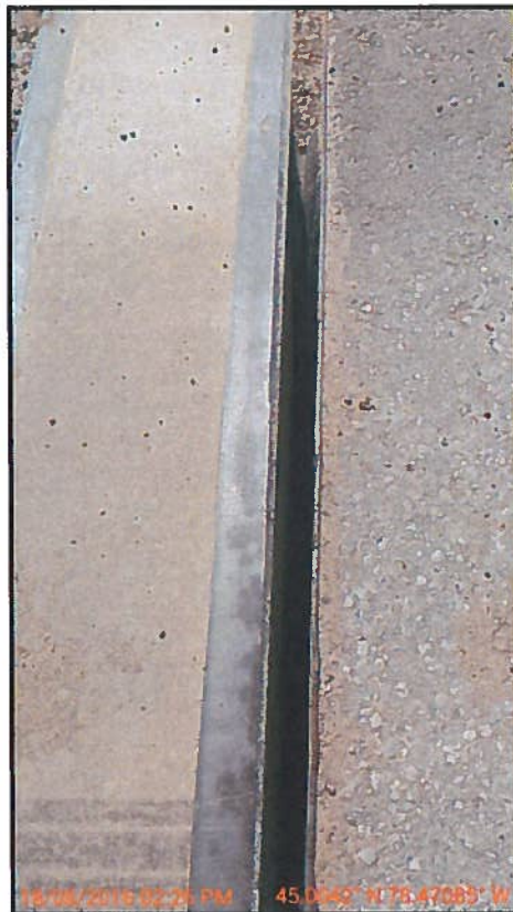
Photo 6 : South Expansion Joint at Deck / Approach Intersection
