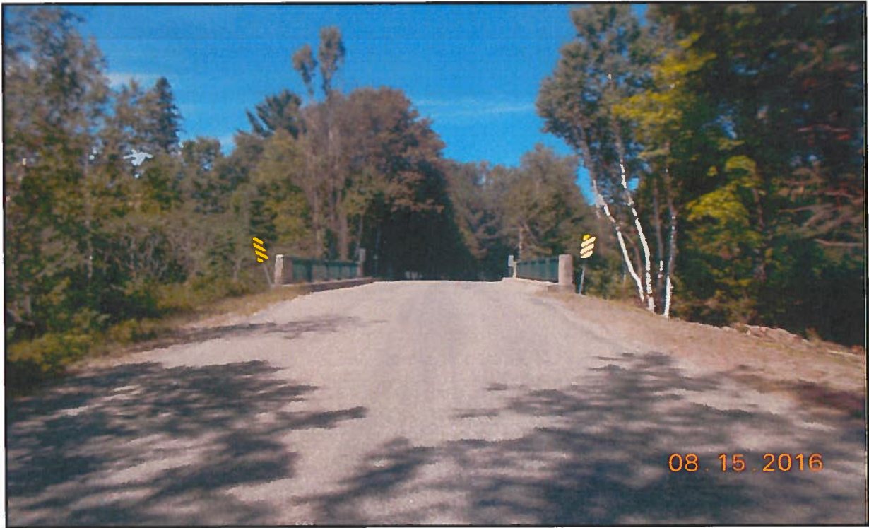
Photo 1 : General Arrangement - Looking West
