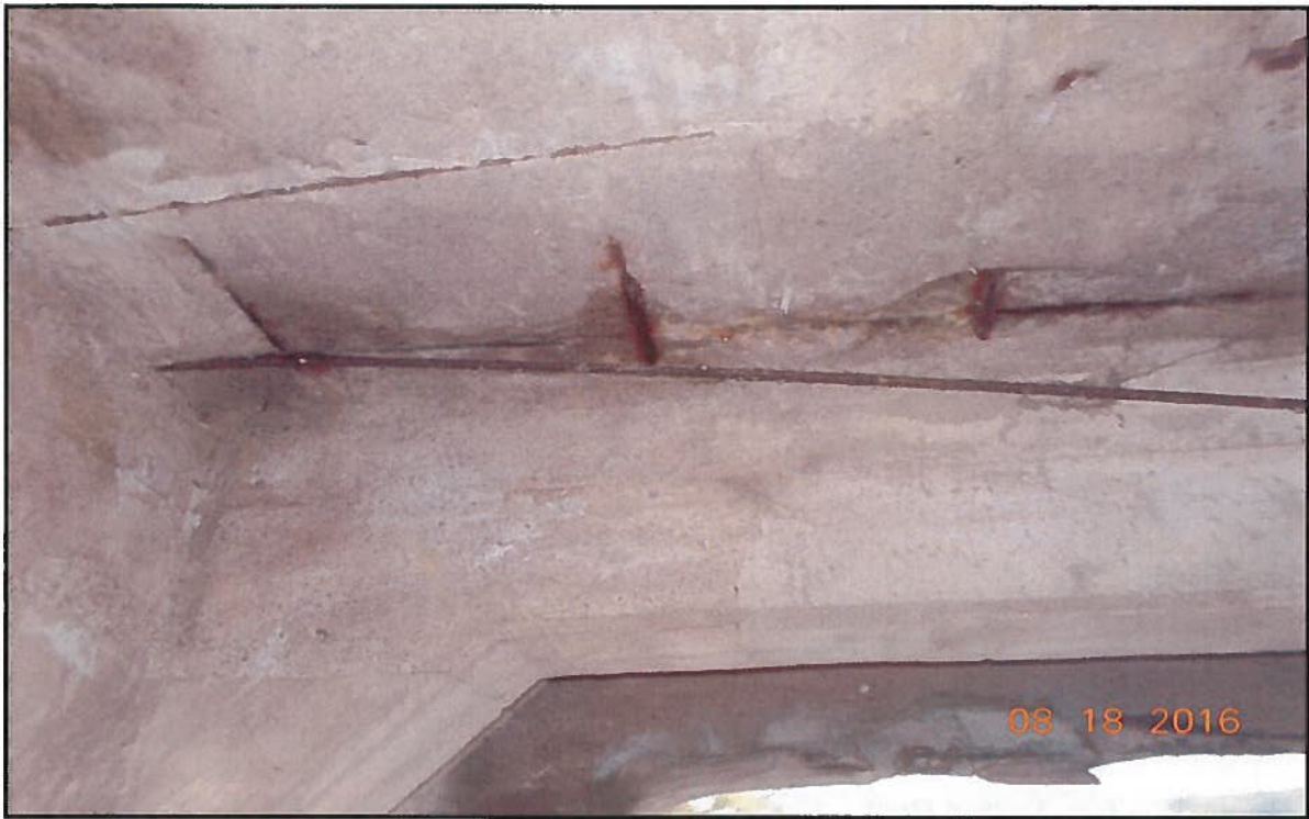
Photo 15 : Int. Soffit at W. Abutment (2 nd Bay From North Face) – Looking North
