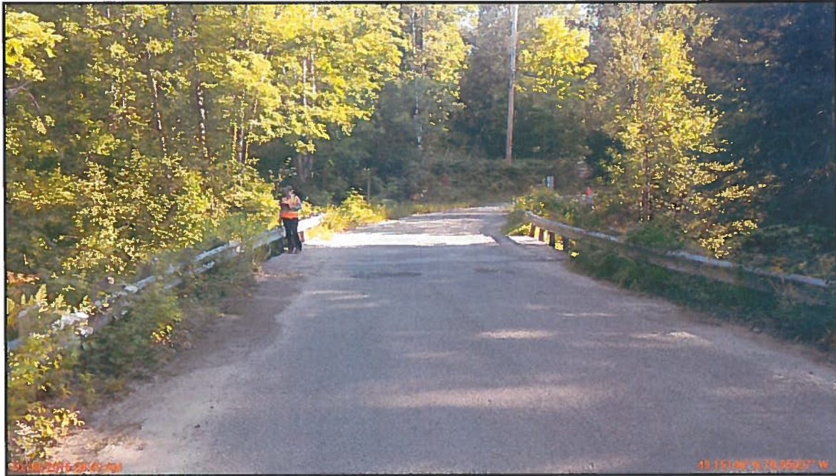
Photo 1 : General Arrangement – Looking North
