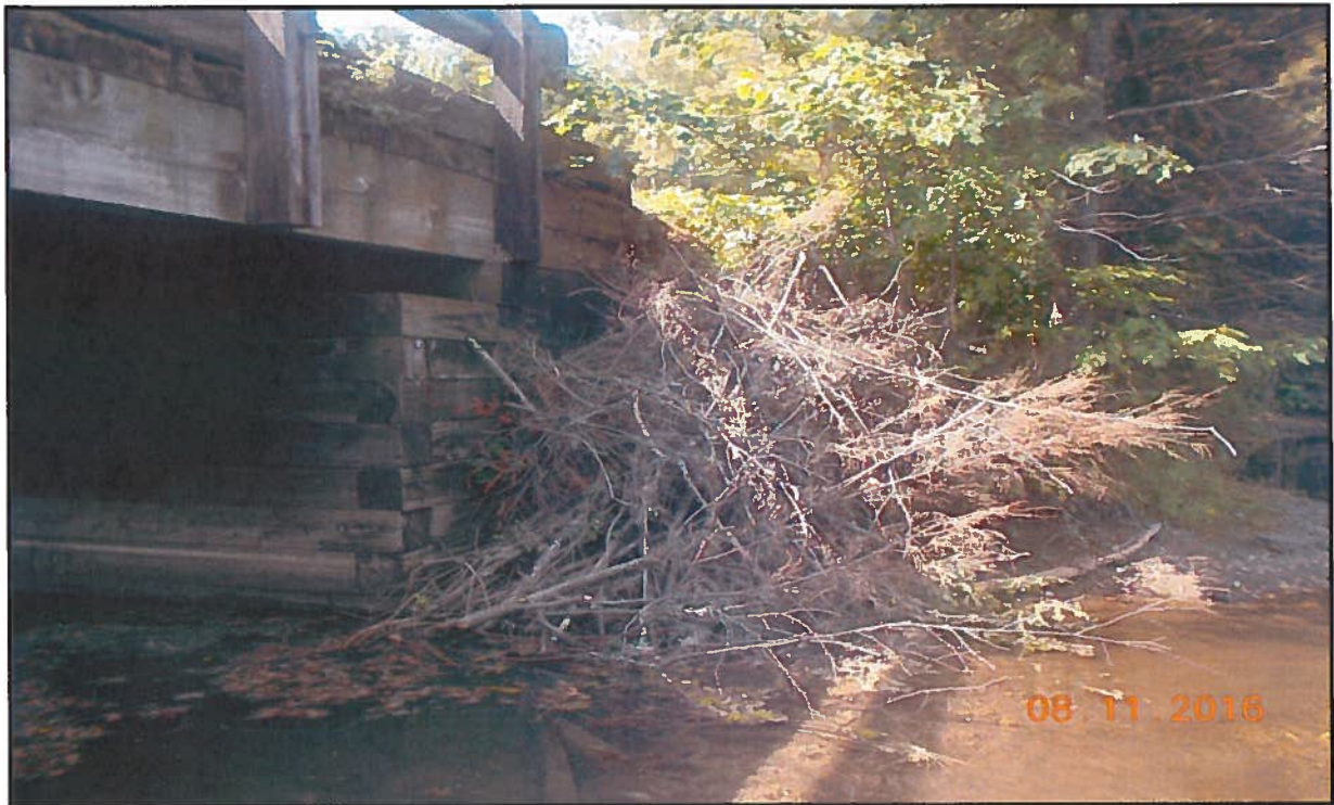
Photo 5 : Southwest Embankment – Looking South
