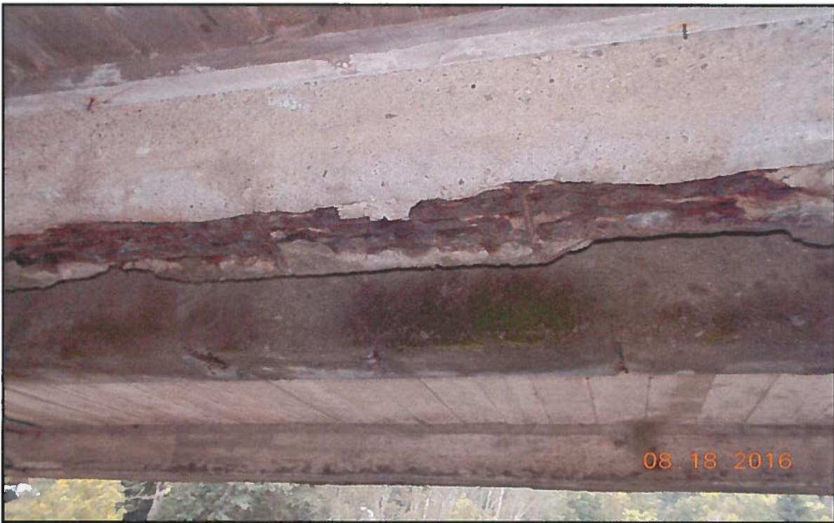
Photo 11 : South Interior Girder (2 nd from End) Mid-Span – Looking South
