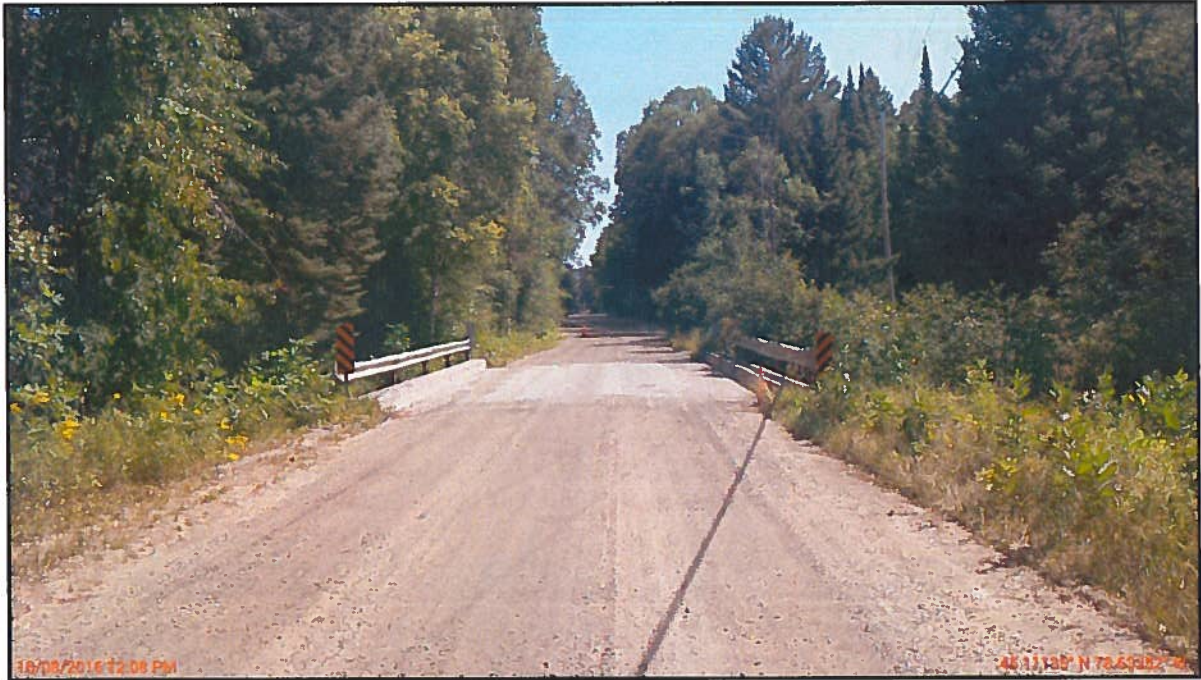
Photo 1 : General Arrangement – Looking East
