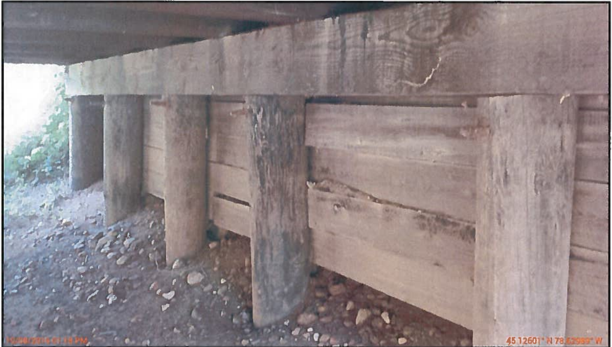
Photo 3: General Arrangement – South Ballast Wall
