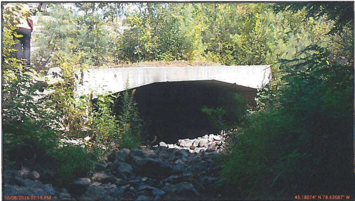
Photo 2: Culvert Outlet - Looking East
