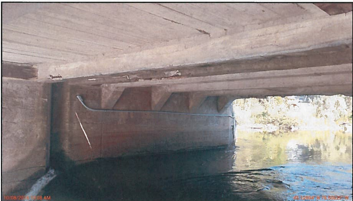
Photo 8 : General Girder Arrangement – Looking Northwest
