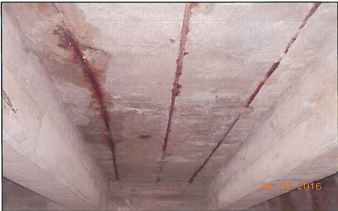
Photo 13 : Interior Soffit (2 nd Bay From North Face) – Looking East
