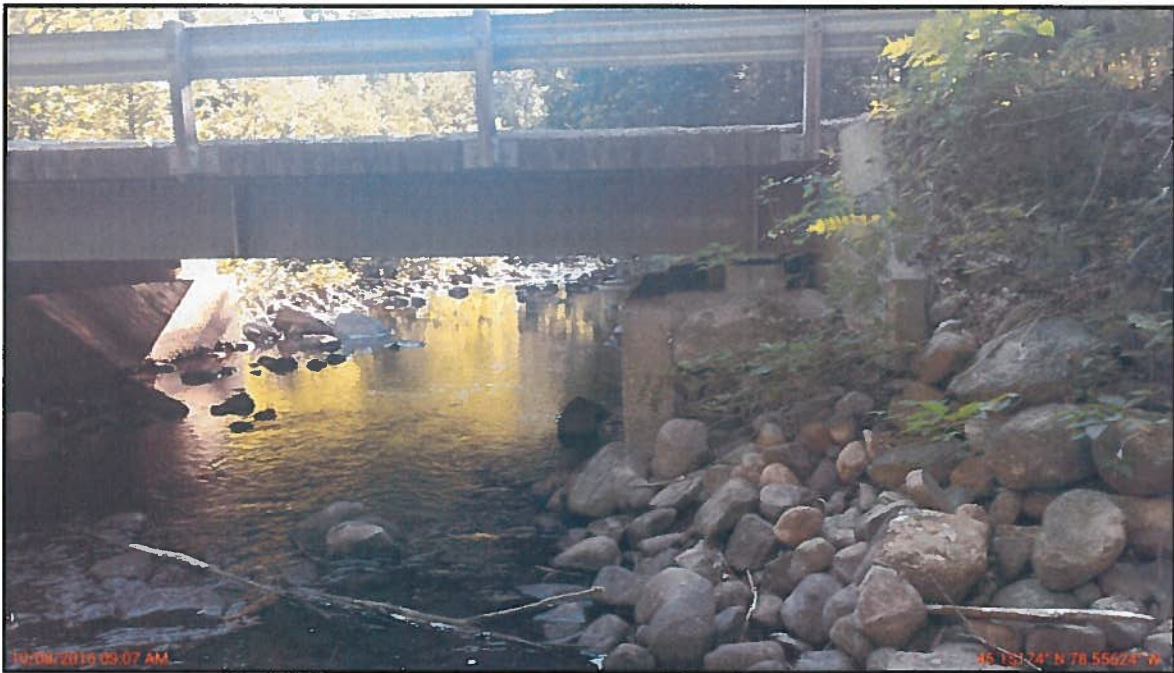
Photo 8 : General Arrangement – Southwest Embankment Looking East
