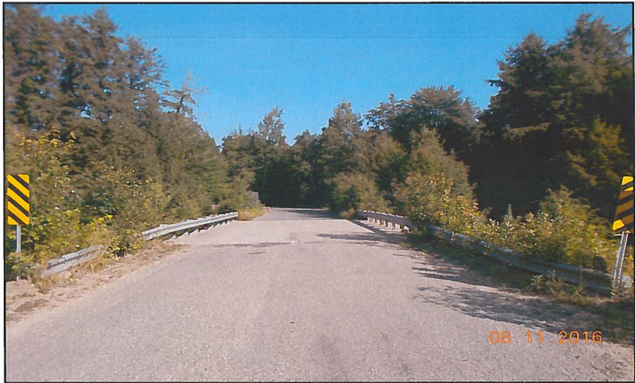
Photo 1 : General Arrangement – Looking North
