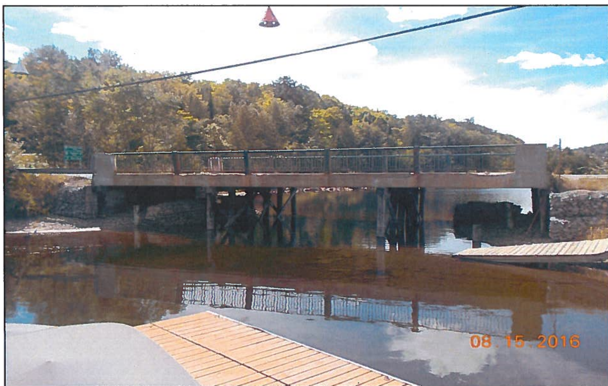
Photo 2 : General Arrangement - Looking West
