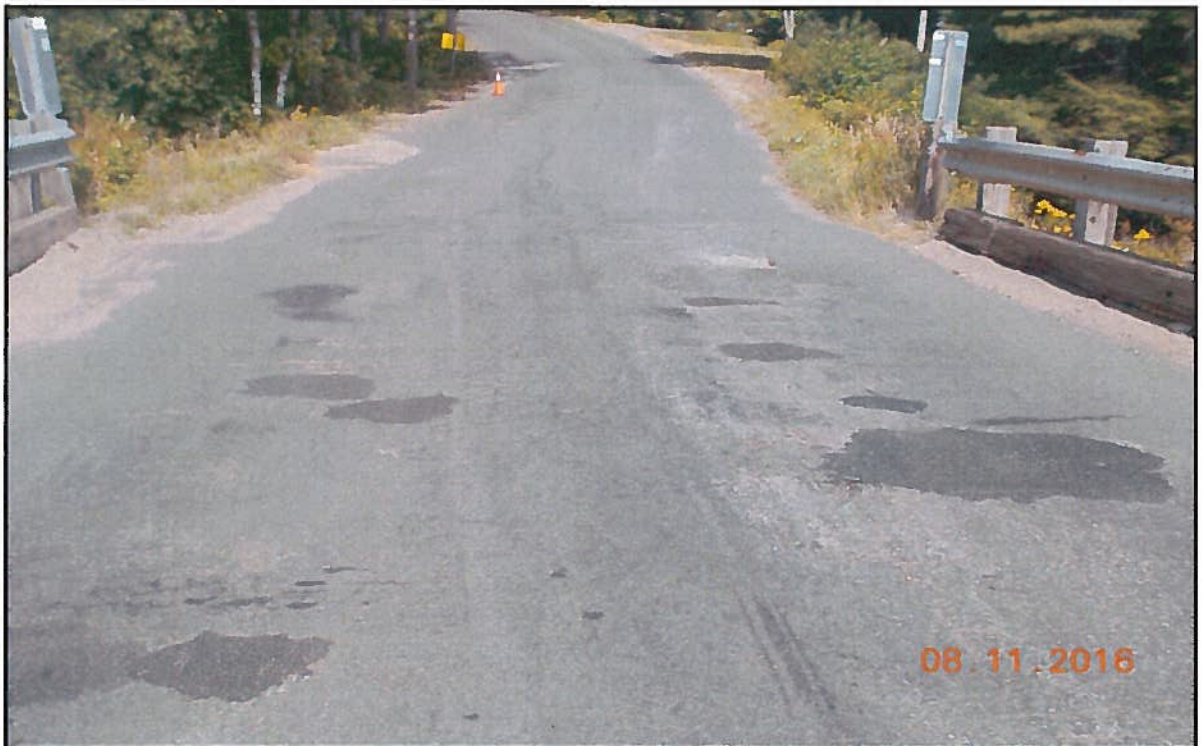
Photo 4: Deck Wearing Surface – Looking West
