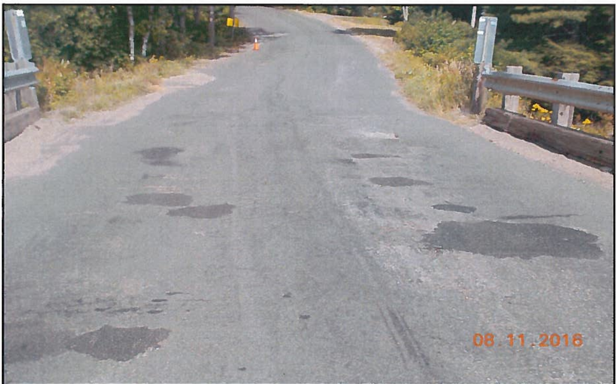
Photo 4: Deck Wearing Surface – Looking West
