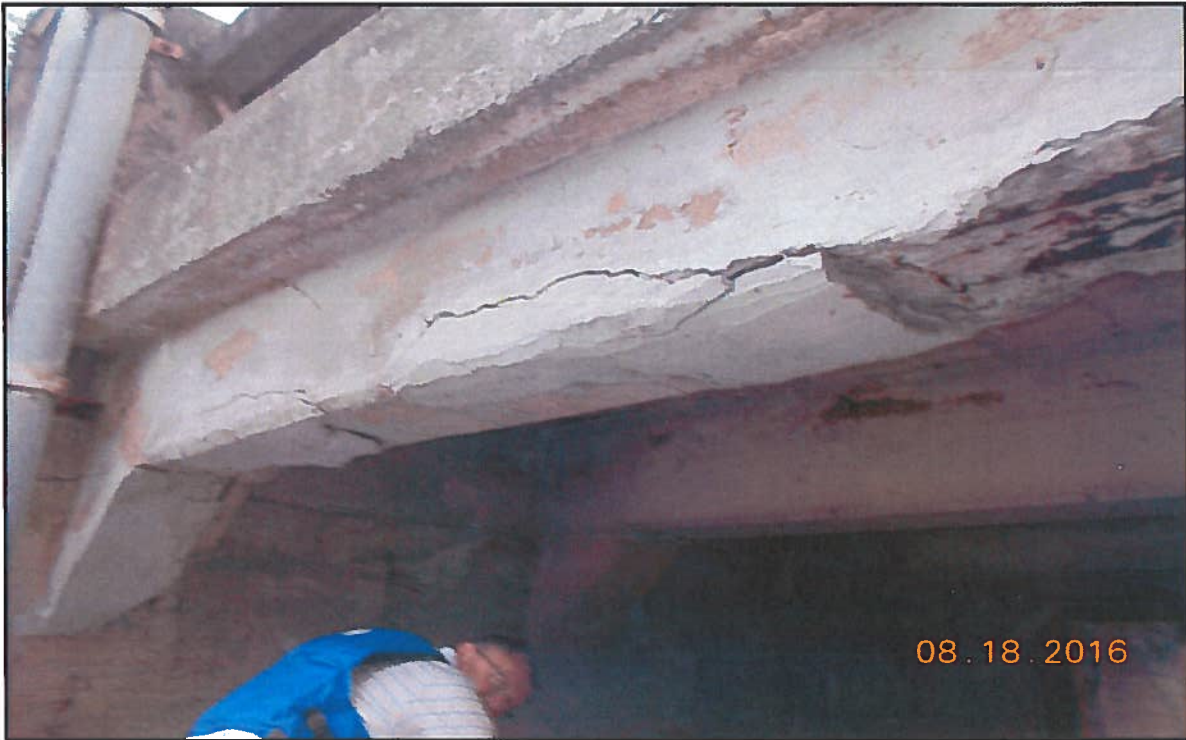
Photo 5 : General View – N. Elevation Exterior Girder at East Abutment
