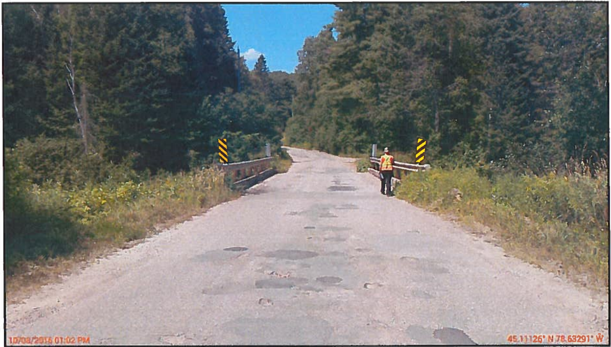
Photo 1: General Arrangement – Looking North
