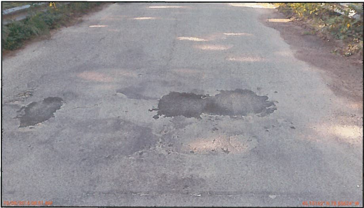
Photo 11 : South Approach Wearing Surface – Looking South
