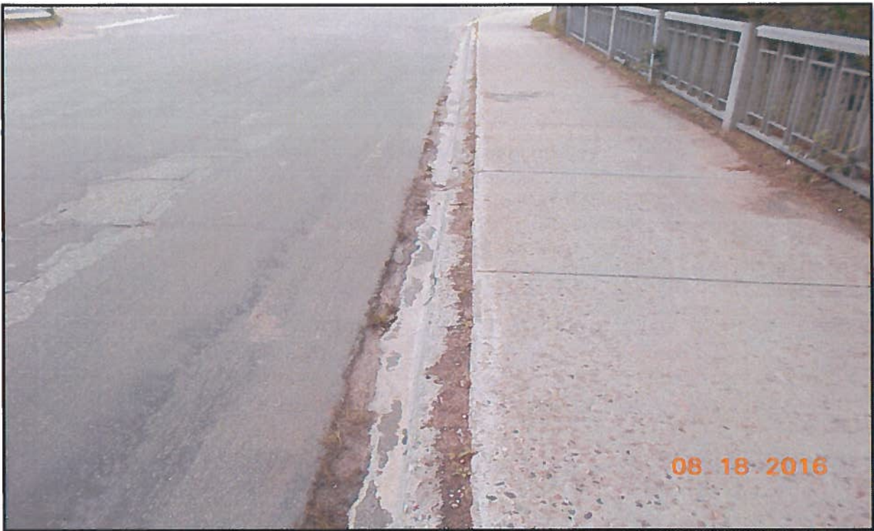
Photo 2 : Edge of Concrete Deck & Curb System - Looking South
