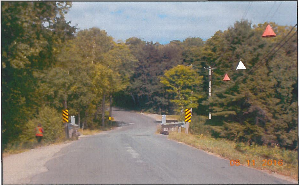
Photo 1: General View – Looking West
