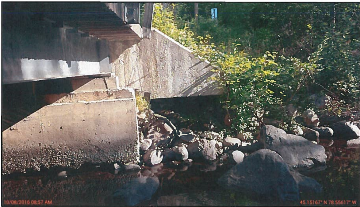
Photo 7 : General Arrangement – Northeast Embankment at Abutment
