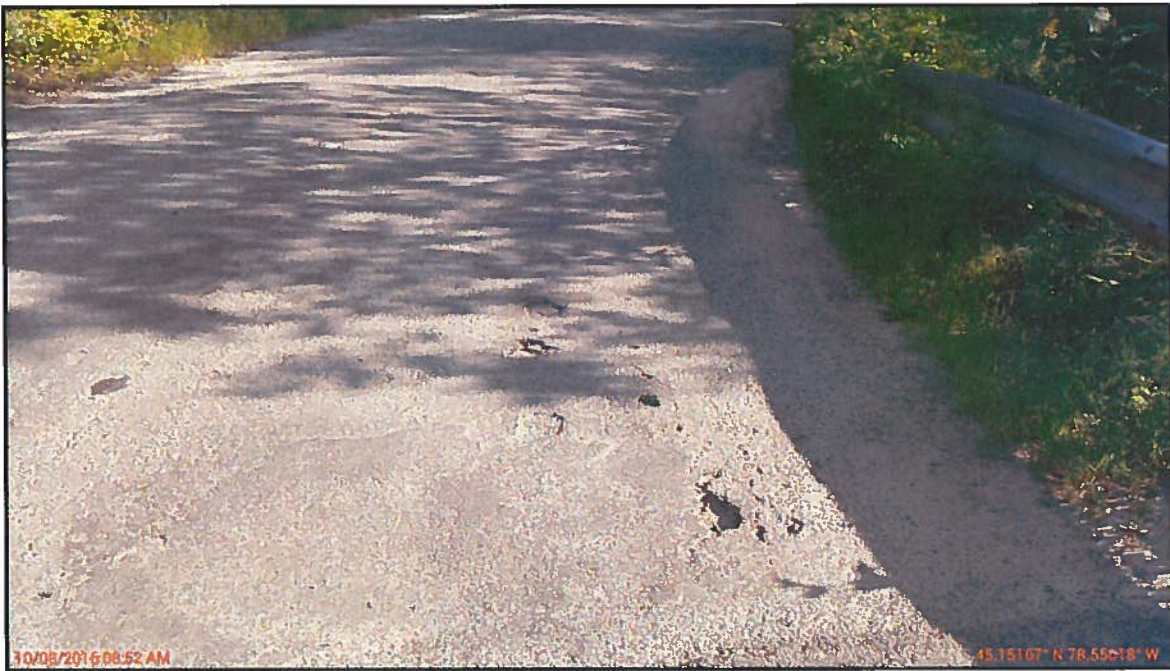
Photo 13 : North Approach Wearing Surface – Looking North
