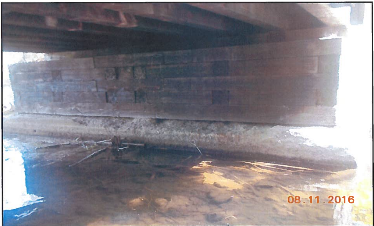
Photo 6 : North Abutment – Looking North
