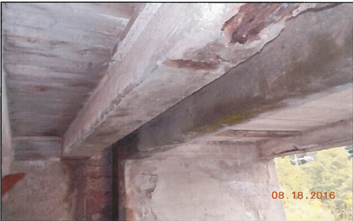
Photo 12 : South Interior Girder (2 nd from End) Mid-Span – Looking Southeast
