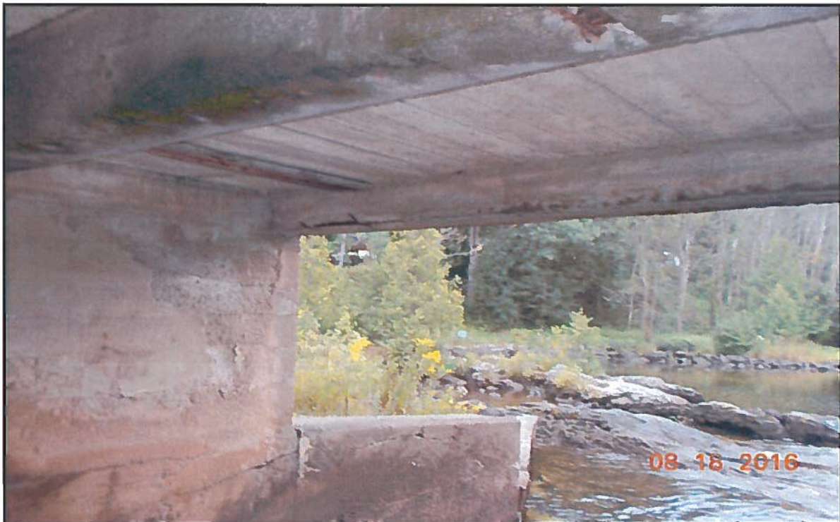
Photo 10 : South Exterior Girder at East Abutment – Looking Southeast
