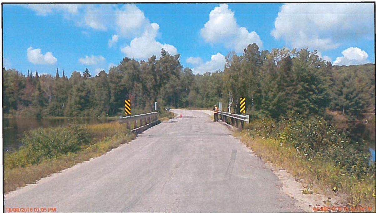
Photo 1 : General Arrangement – Looking North
