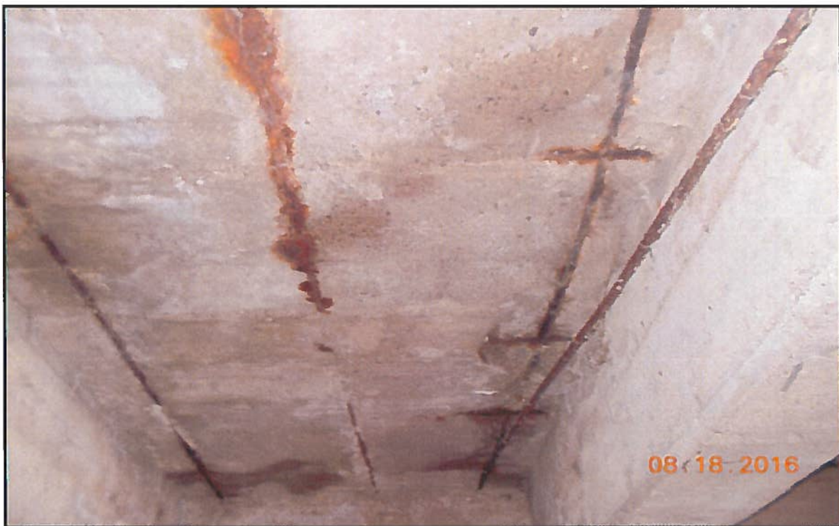
Photo 14 : Interior Soffit (2 nd Bay From North Face) – Looking West
