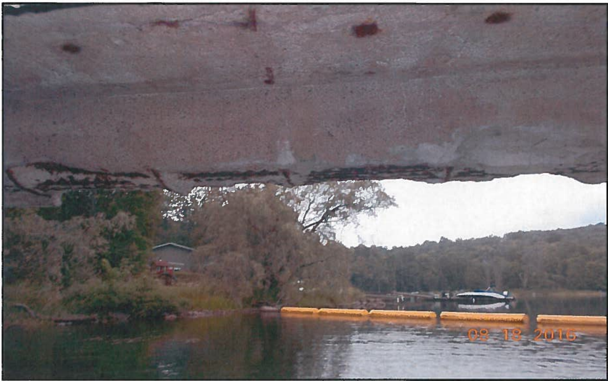
Photo 7 : North Exterior Girder at Mid Span – Looking North
