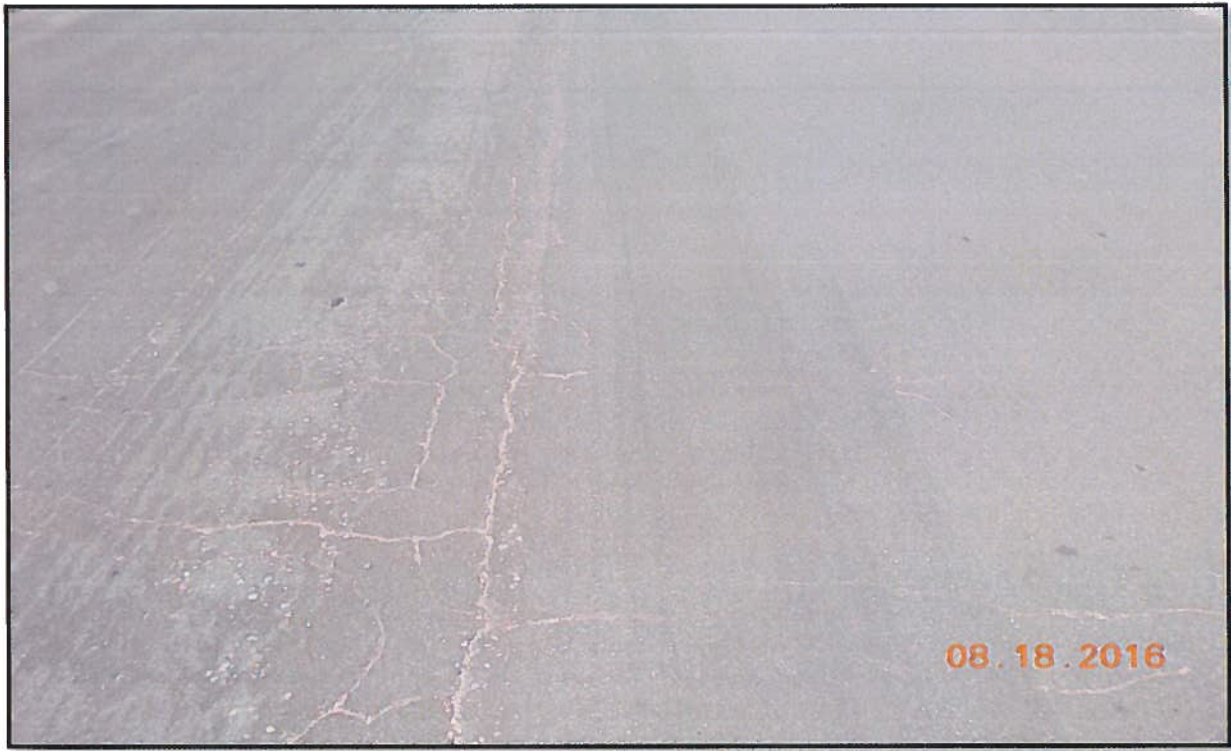
Photo 1 : Deck Wearing Surface - Looking South
