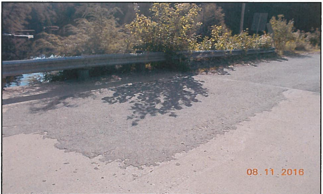
Photo 4 : Deck Wearing Surface – Asphalt Patching
