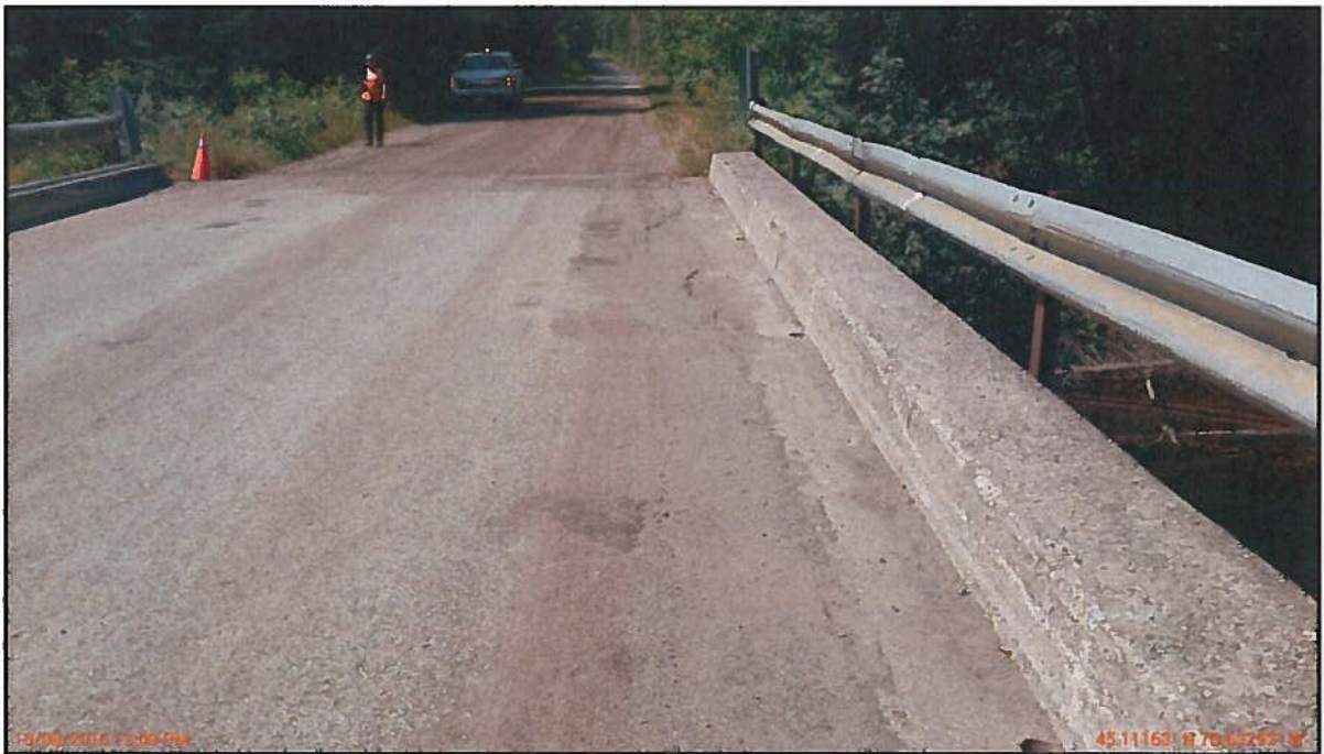
Photo 4: Deck Wearing Surface – Looking West
