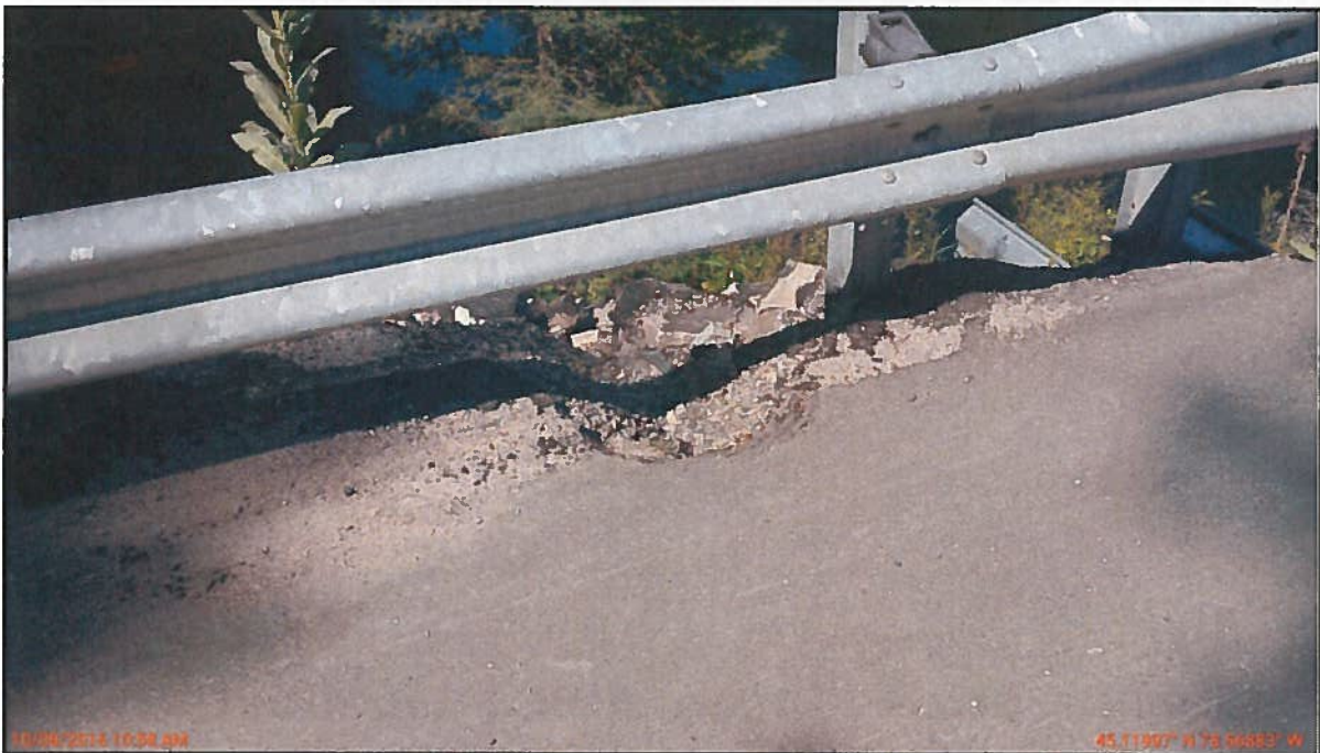
Photo 4 : Asphalt Wearing Surface Edge of Pavement – Southwest Quadrant
