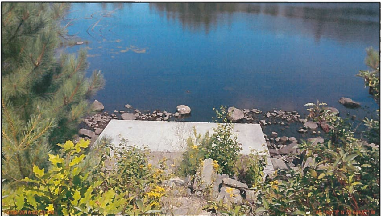
Photo 4: General View Culvert Inlet – Looking East
