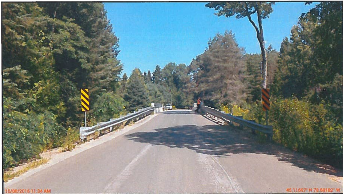
Photo 2 : General Arrangement – Looking North
