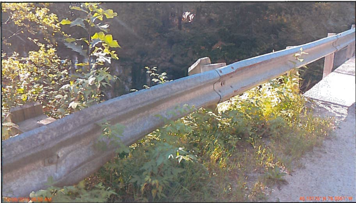
Photo 14 : Approach Guiderail – Northeast Quadrant
