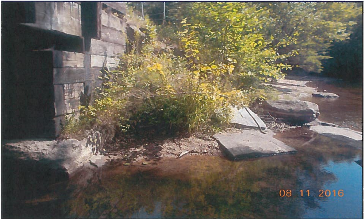
Photo 3 : Northeast Embankment – Looking North
