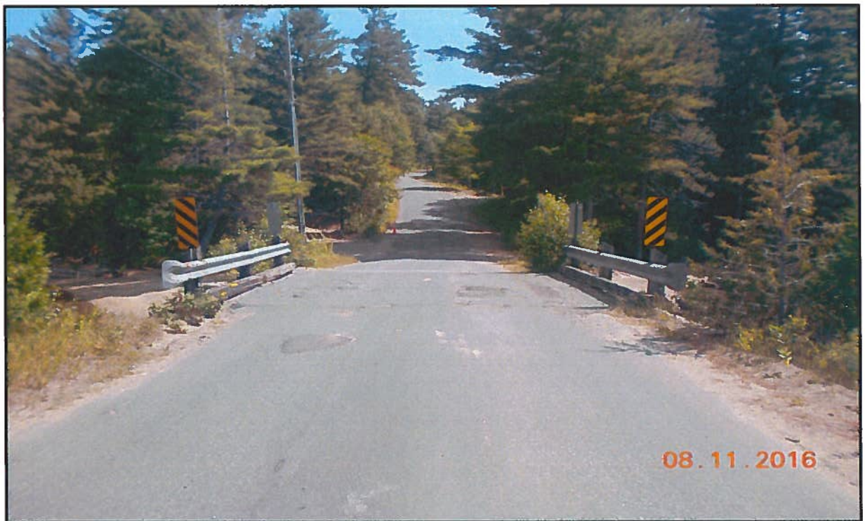
Photo 2: General Arrangement – Looking East
