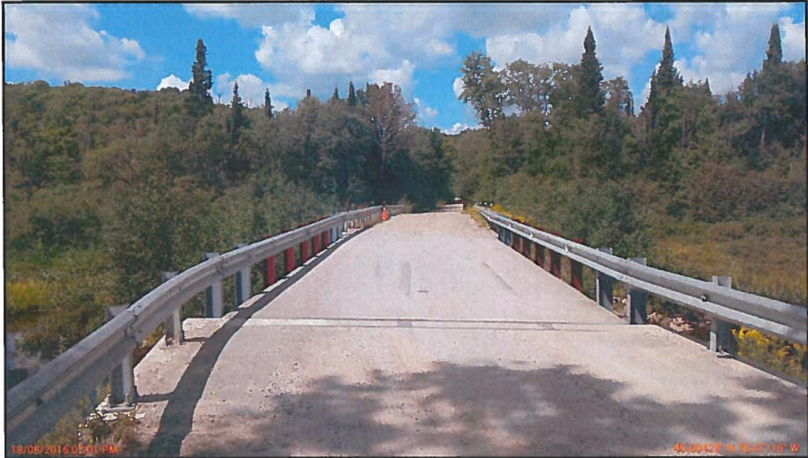
Photo 1 : General Arrangement – Looking North
