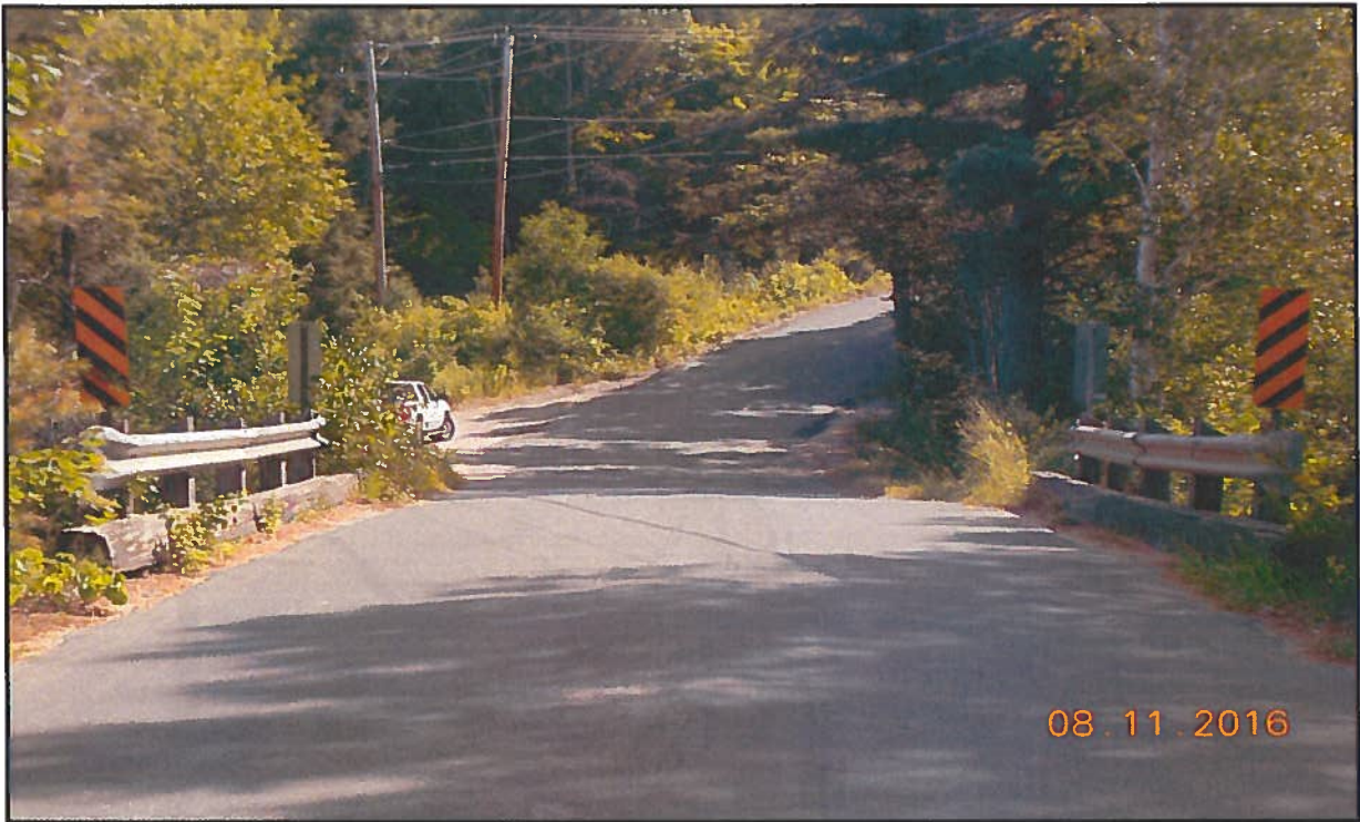
Photo 1 : General Arrangement – Looking North
