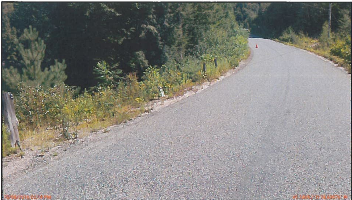
Photo 6: Typical Guide Rail System & Wearing Surface – Looking Southwest
