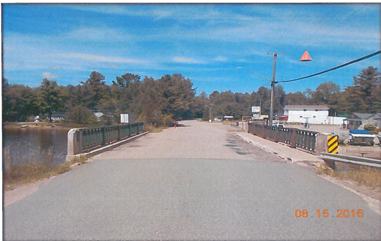
Photo 1 : General Arrangement - Looking North
