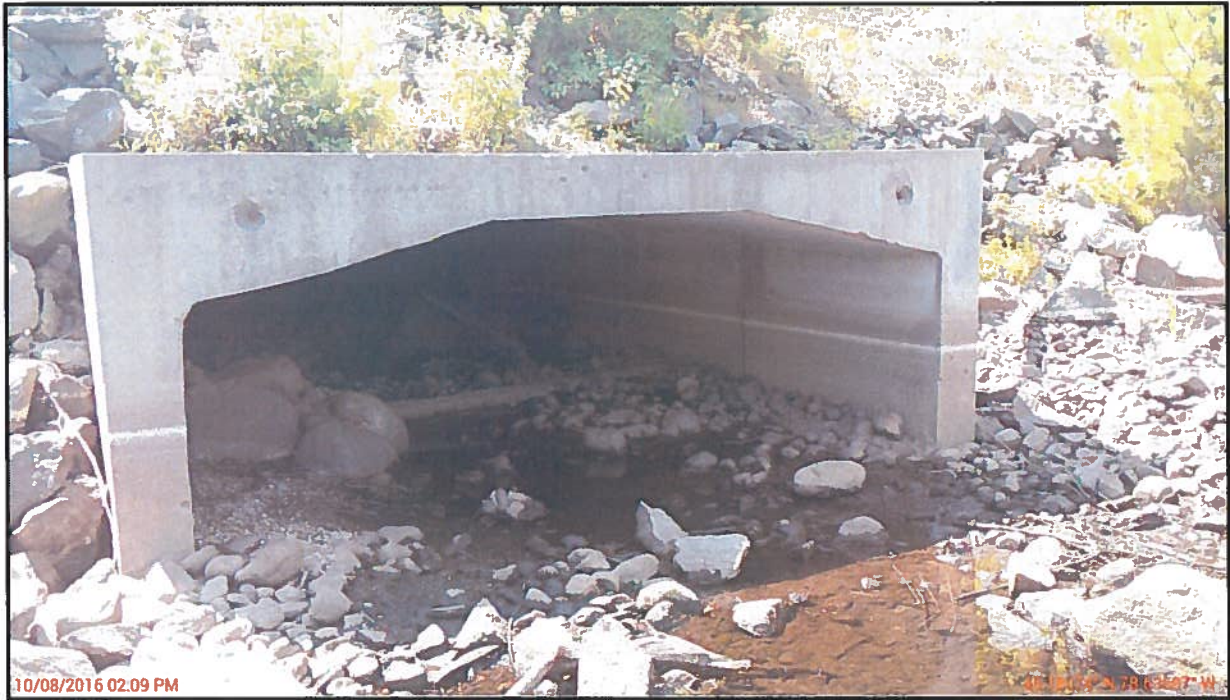
Photo 1: Culvert Inlet - Looking West
