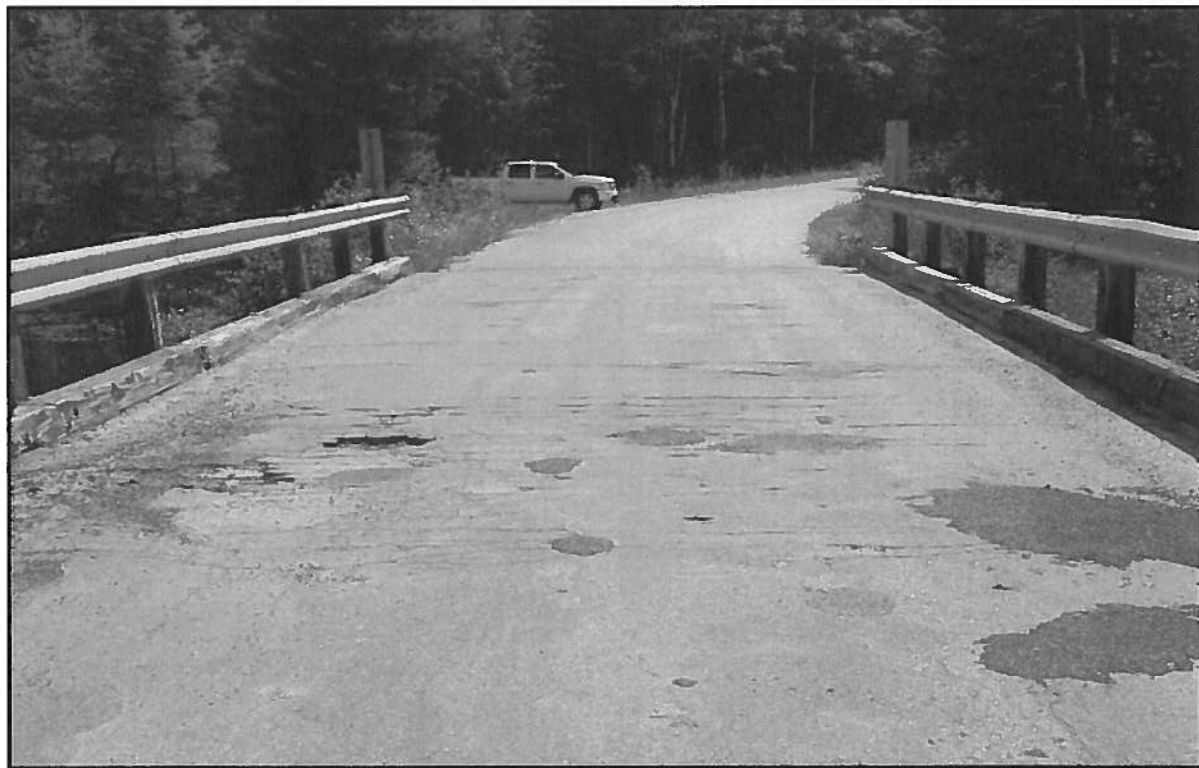
Photo 4 : General Arrangement – Deck Wearing Surface Looking South
