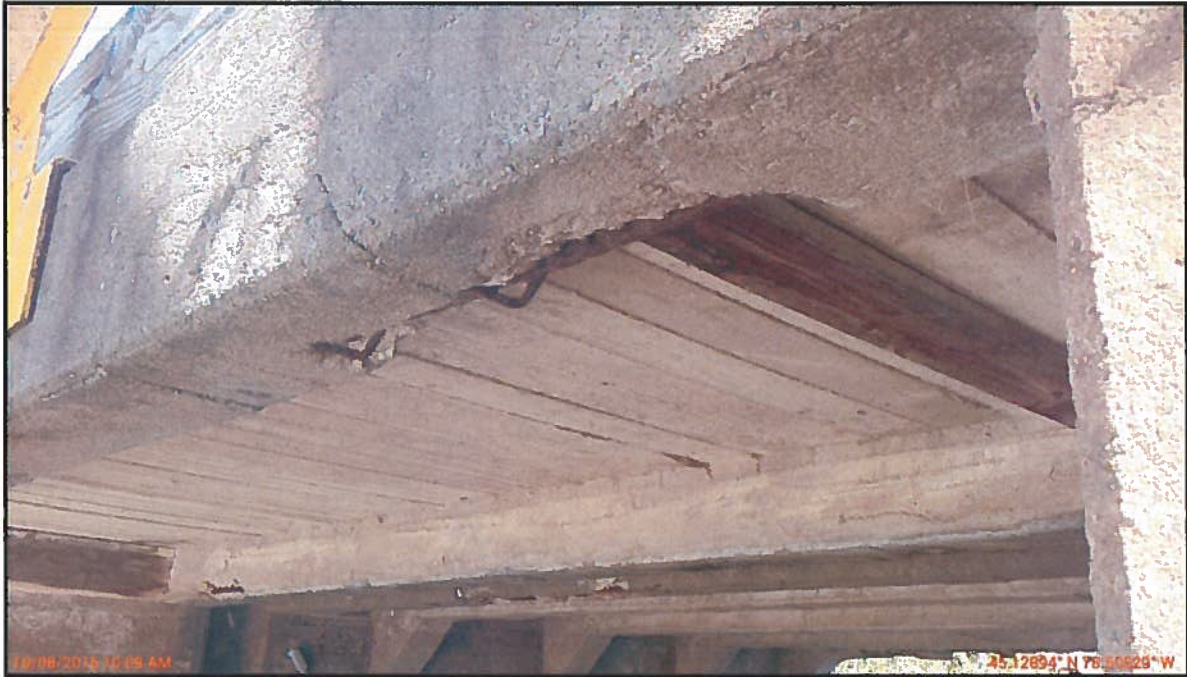
Photo 9 : South Exterior Girder at East Abutment – Looking Northwest
