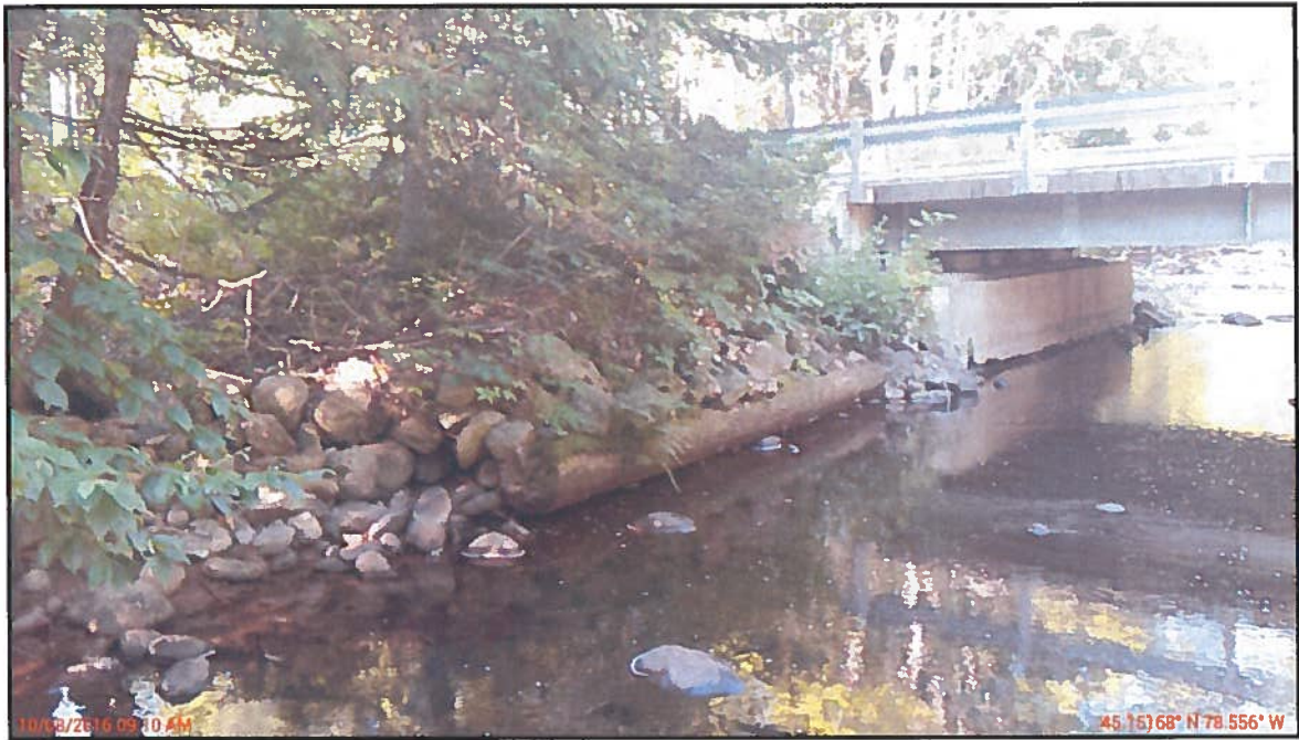
Photo 5 : General Arrangement – Southeast Embankment
