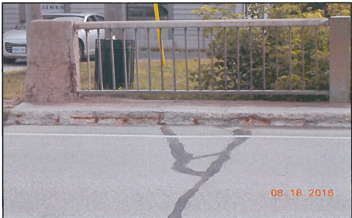
Photo 6 : Curb / Sidewalk and Railing System / End Post – Northeast Quadrant
