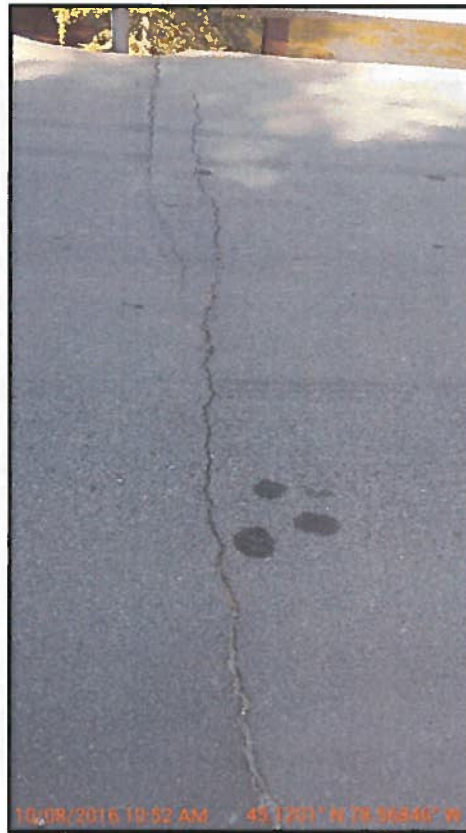
Photo 3 : South Approach Wearing Surface
