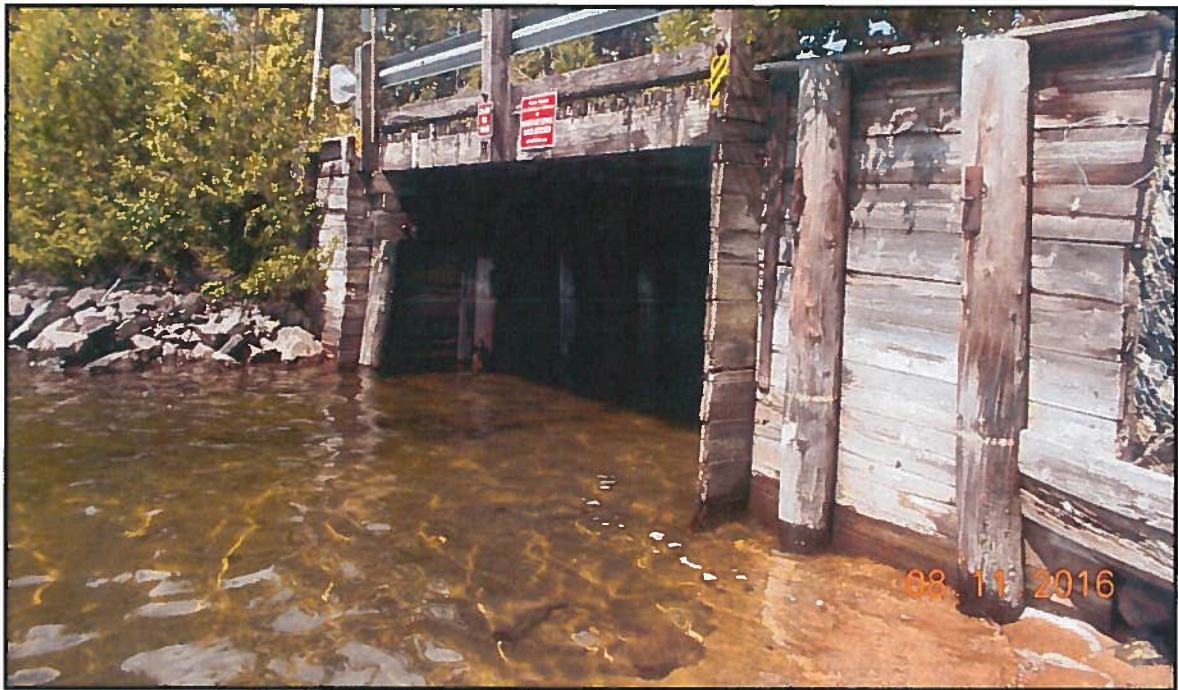
Photo 3: General Arrangement – Southeast Elevation
