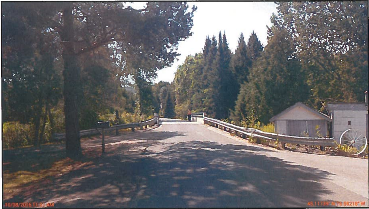
Photo 1 : General Arrangement – Looking South
