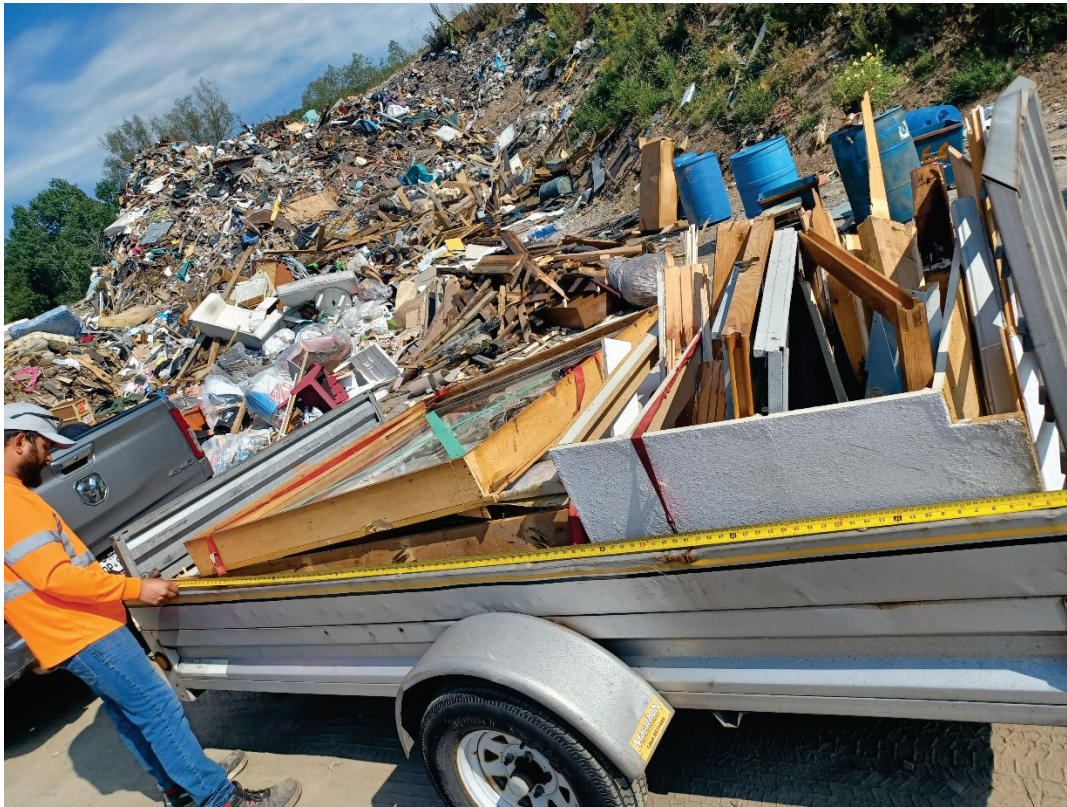
Figure 1.1 Measuring the length, width, and height of the trailer to determine the volume of CND material being disposed of.
