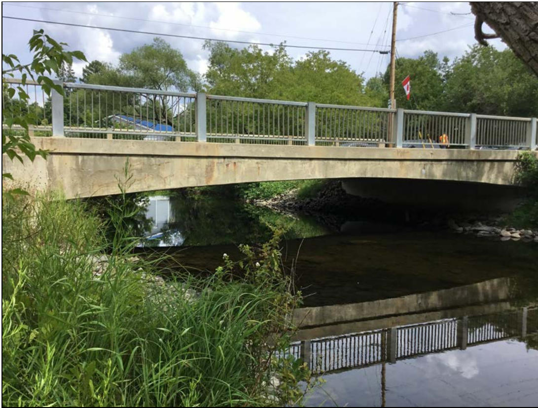
Description: General elevation, west.
