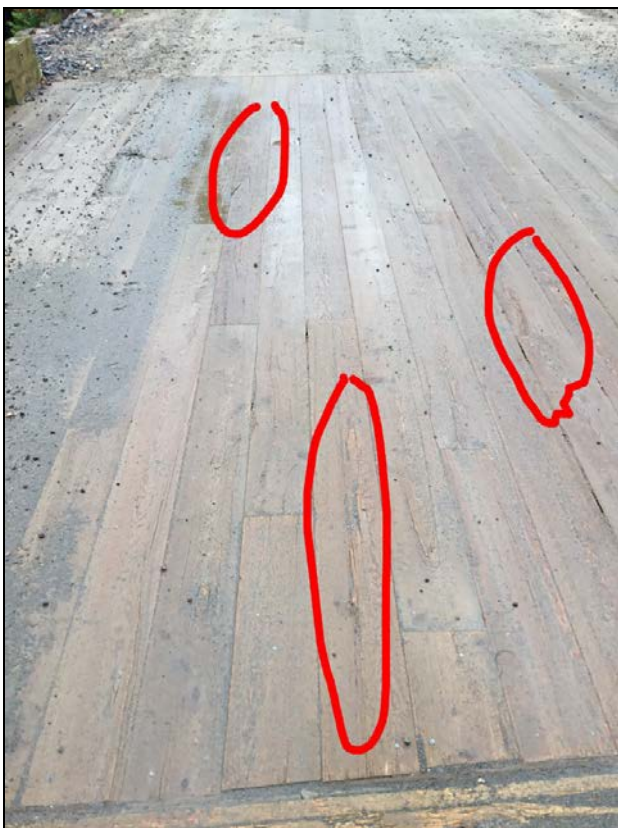
Description: Light checks on deck wearing surface.
