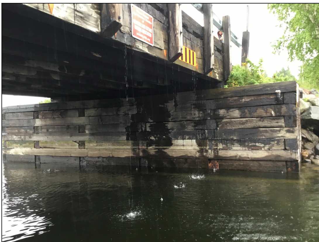
Description: East abutment (typical condition).
