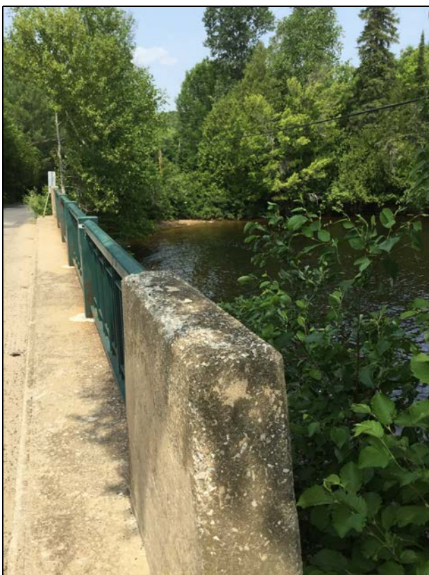
Description: Northeast parapet
