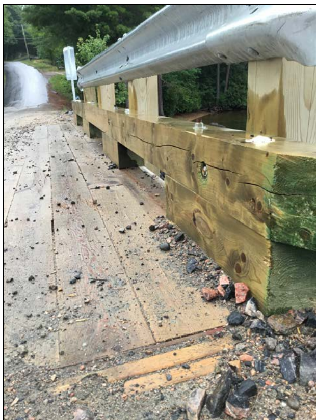
Description: Southwest corner of curb system. Sidewalks/Curbs / Curbs (North and South)
