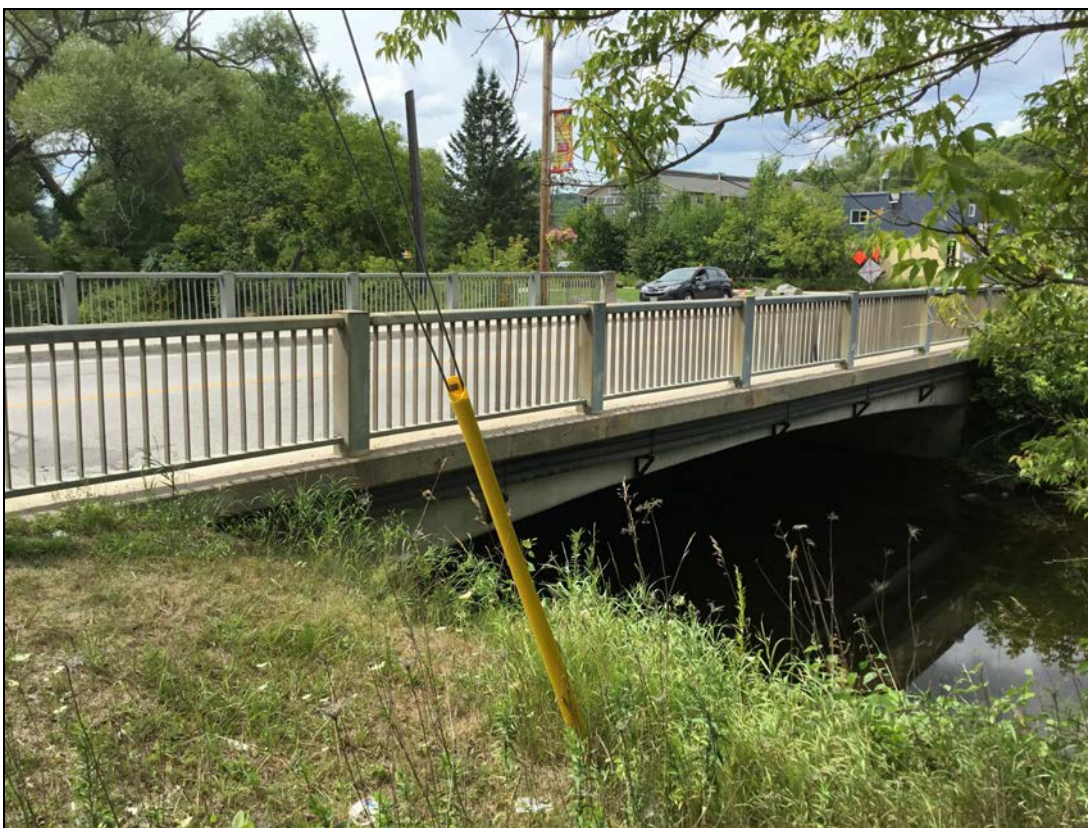
Description: General elevation, east.
