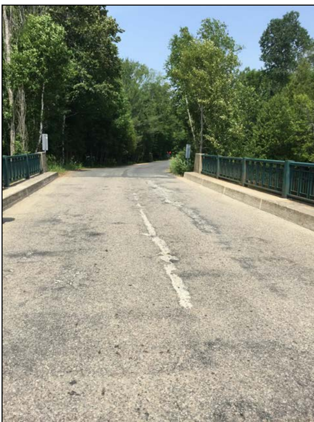
Description: Wearing surface looking east Decks / Wearing Surface (Top)
