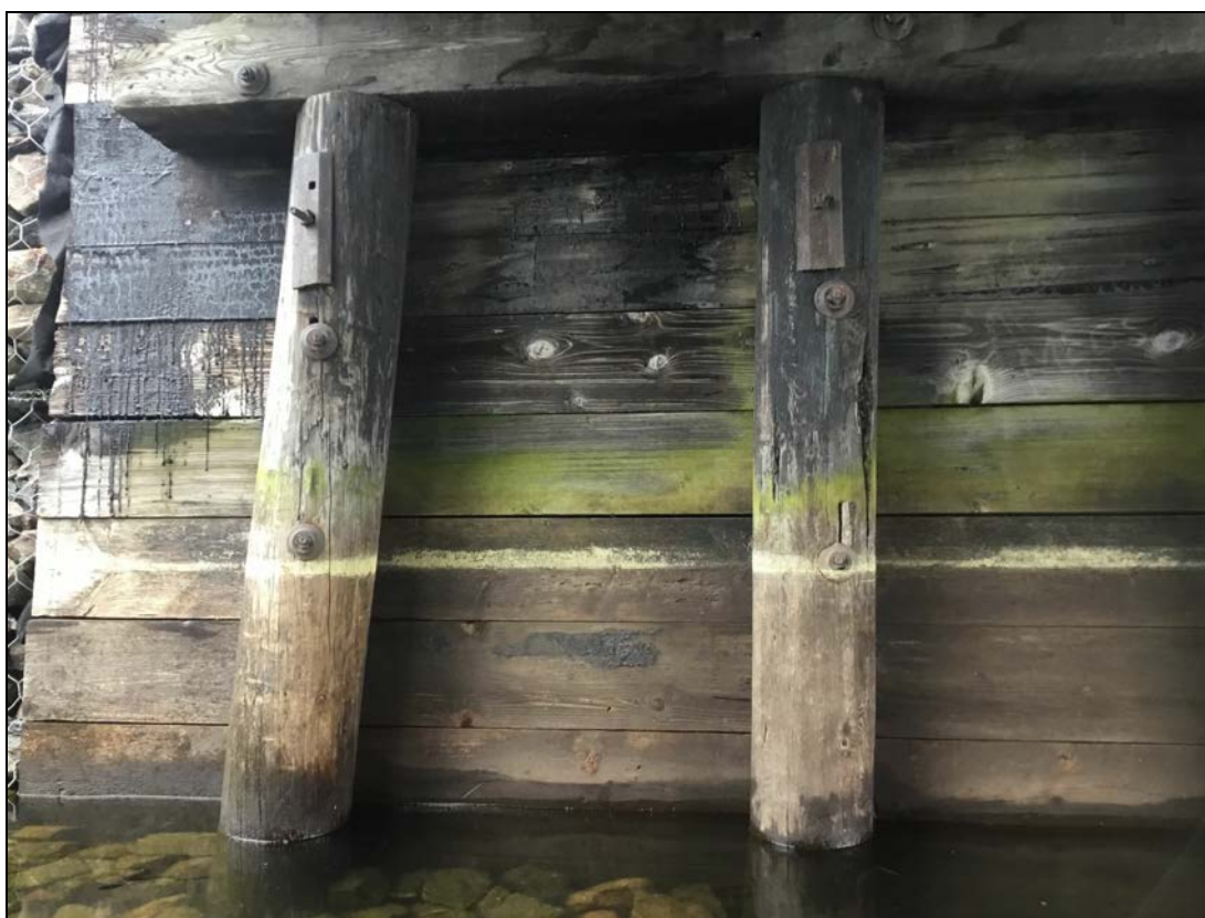
Description: East wall #1, northeast quadrant. High water level visible. Abutments / Ballast Walls (East and West)
