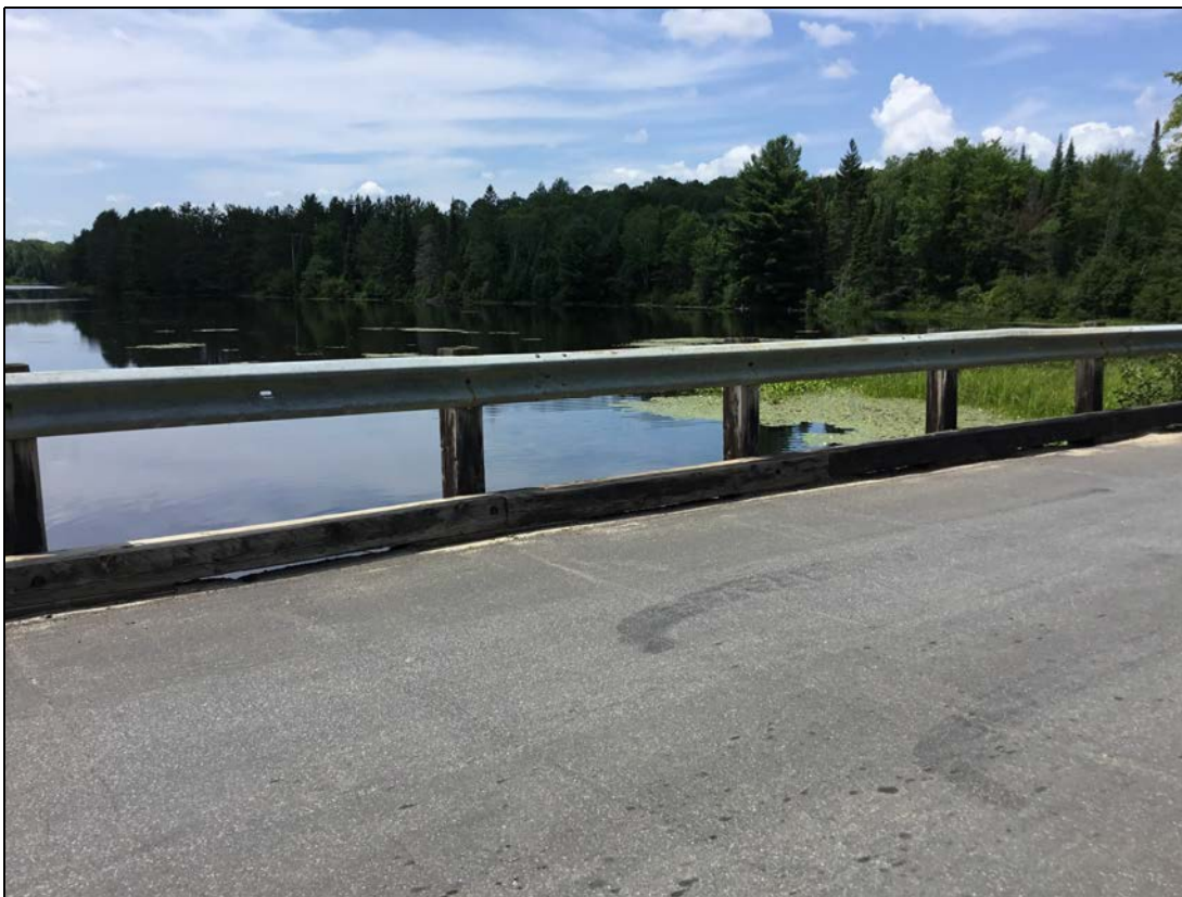
Description: Original curb, typical condition. Sidewalks/Curb / Curb (N /S)
