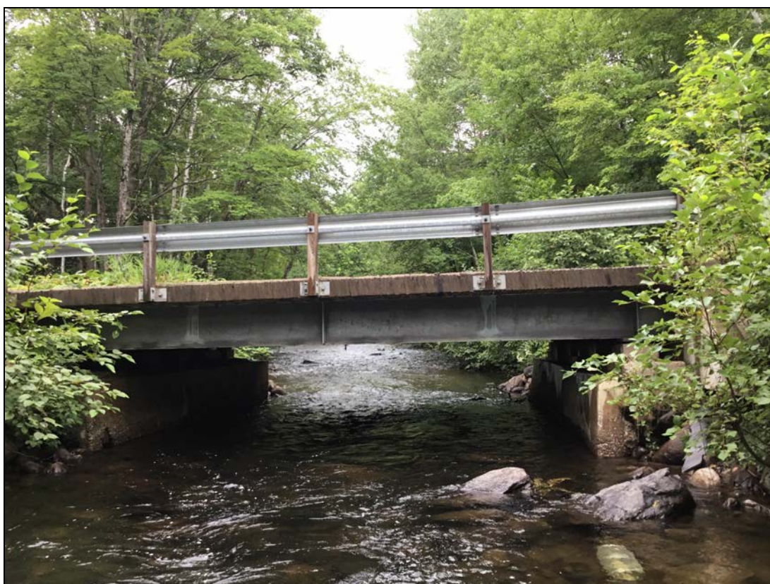
Description: General elevation, east.
