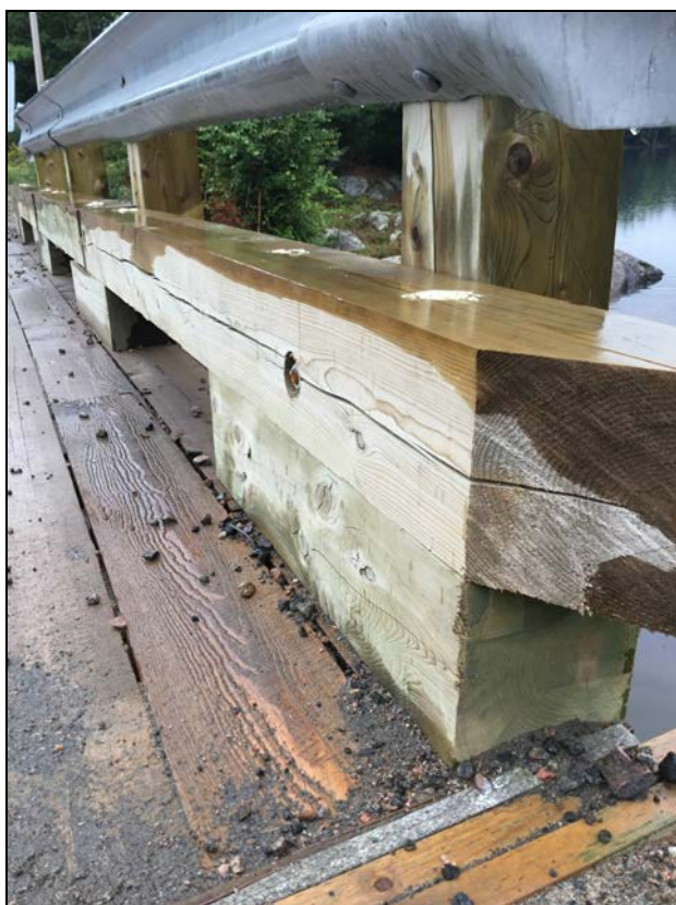
Description: Northeast corner of curb system. Sidewalks/Curbs / Curbs (North and South)
