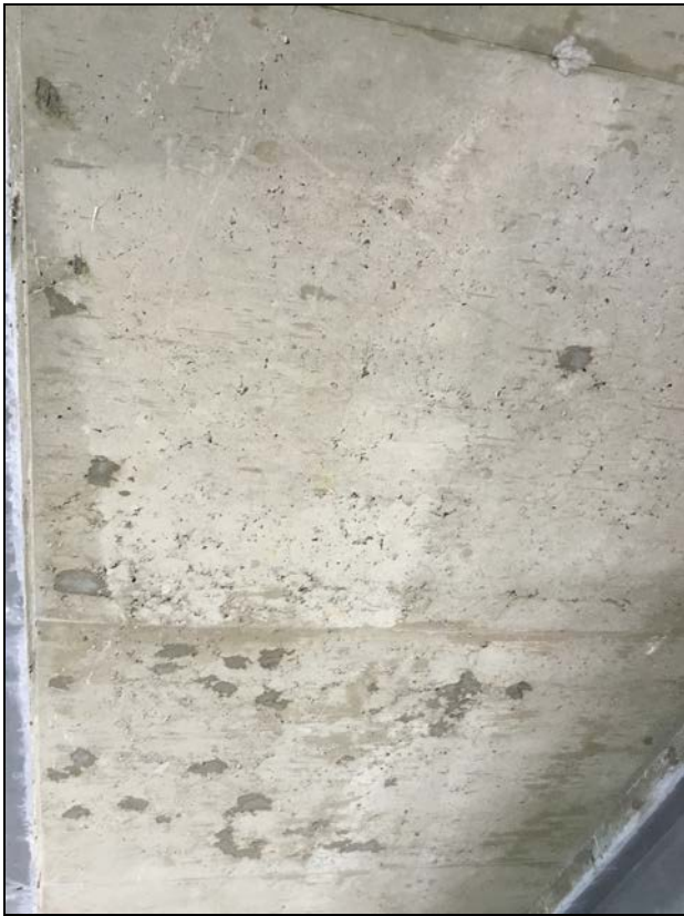
Decks / Soffit - Thin Slab
