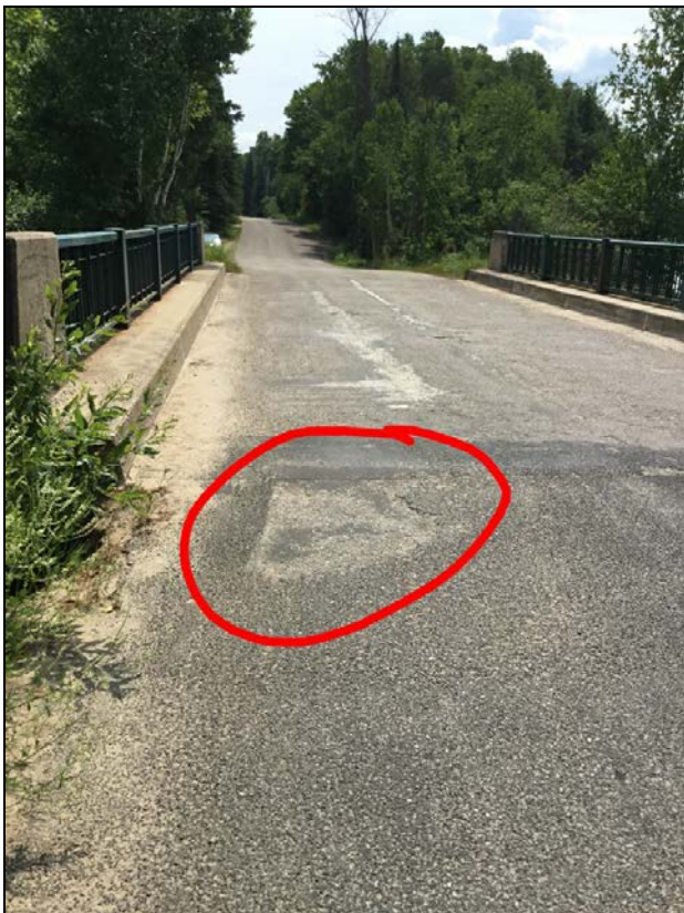
Description: North side of west approach Approaches / Wearing Surface (East and West)
