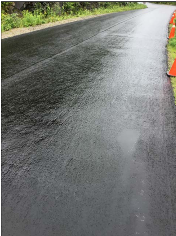
Description: West approach wearing surface, general condition.
