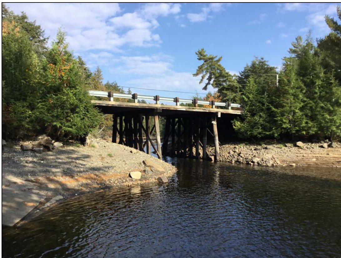
Description: General elevation, looking east.
