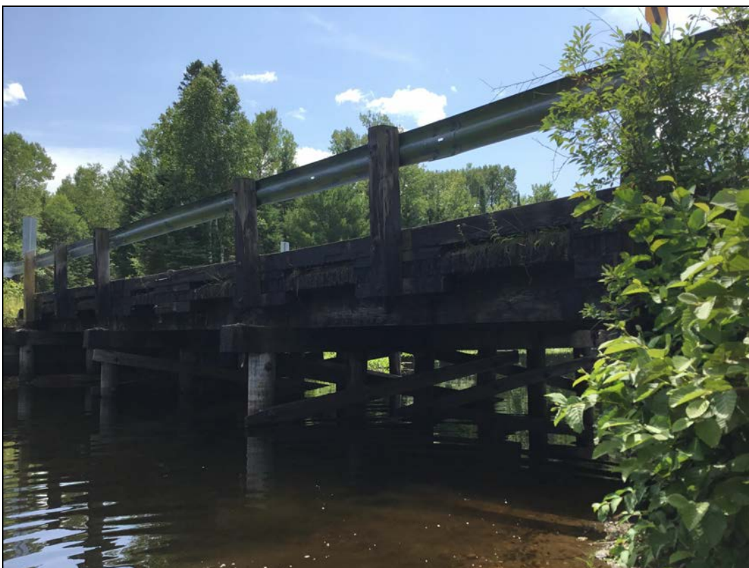
Description: General elevation, west.
