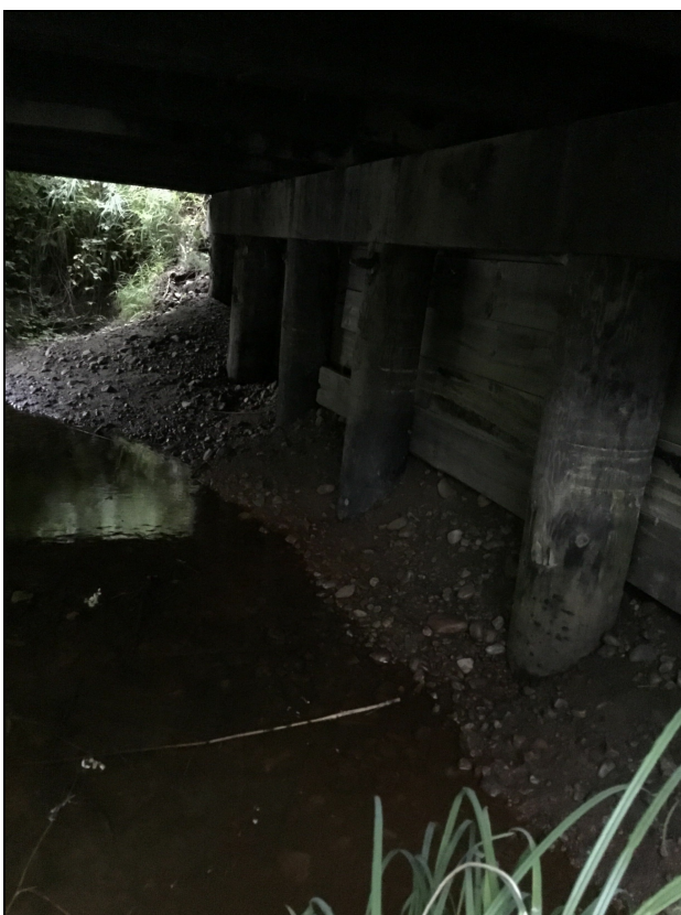
Description: West ballast wall.
