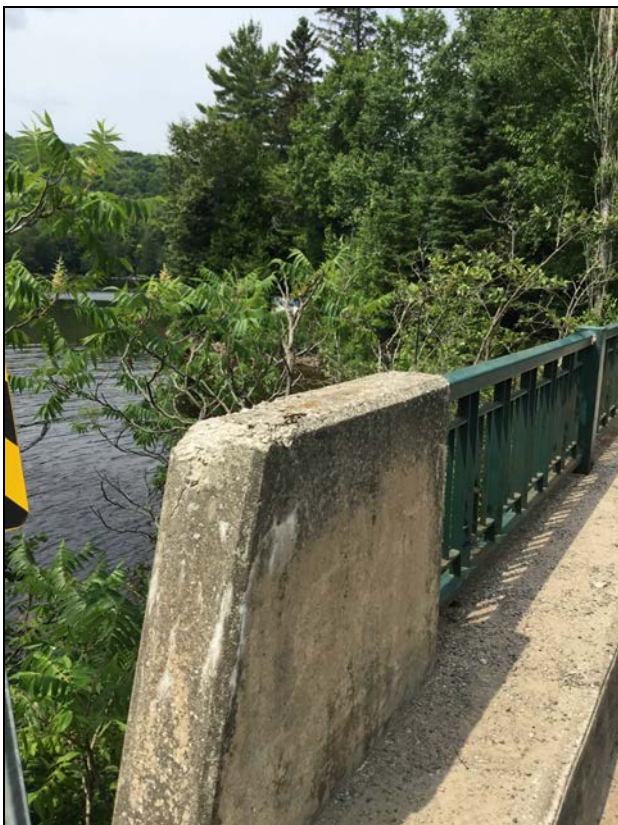
Description: Southeast parapet
