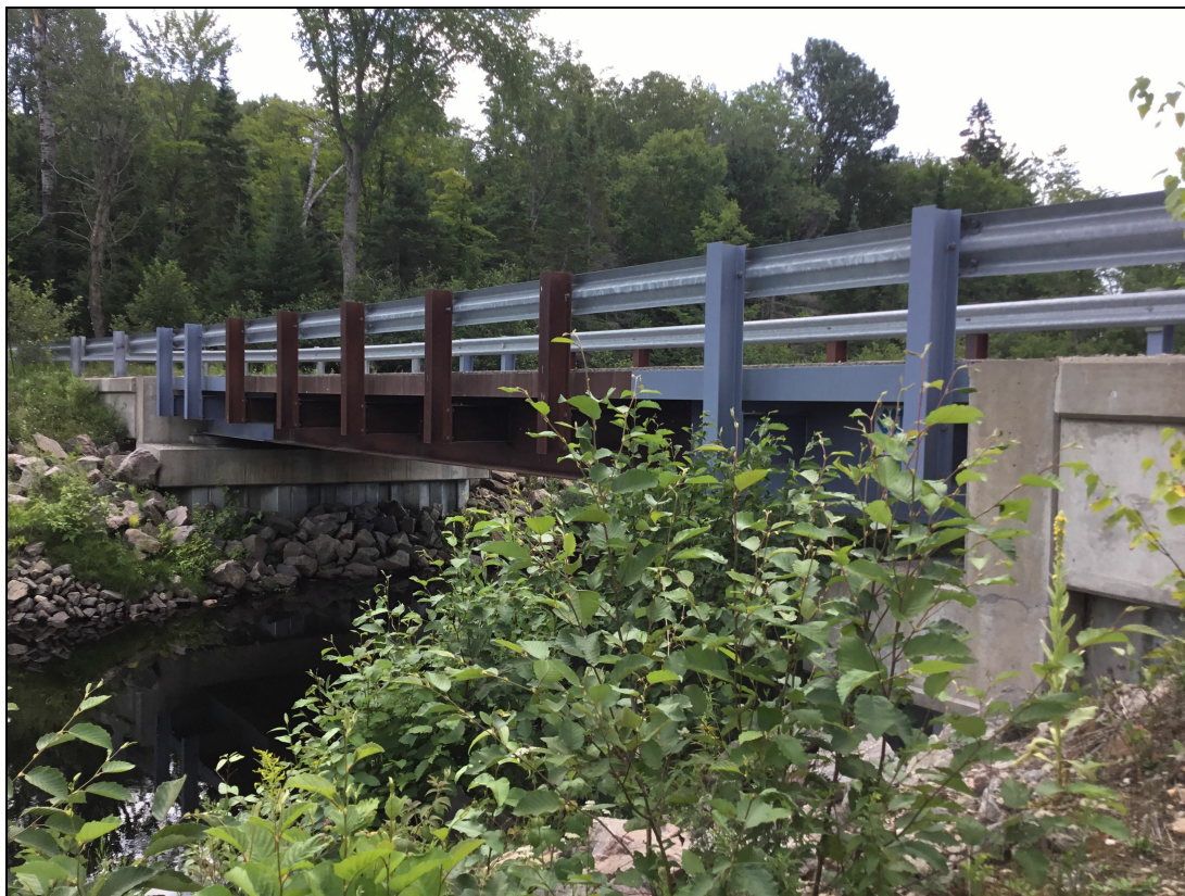
Description: General elevation, east.
