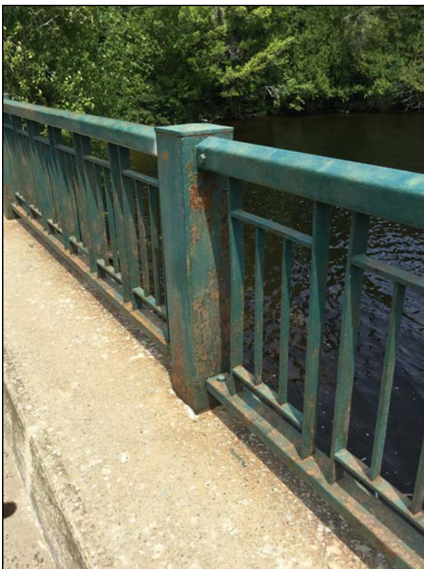
Description: North side, second post from the west Barriers / Hand Railings (North and South)
