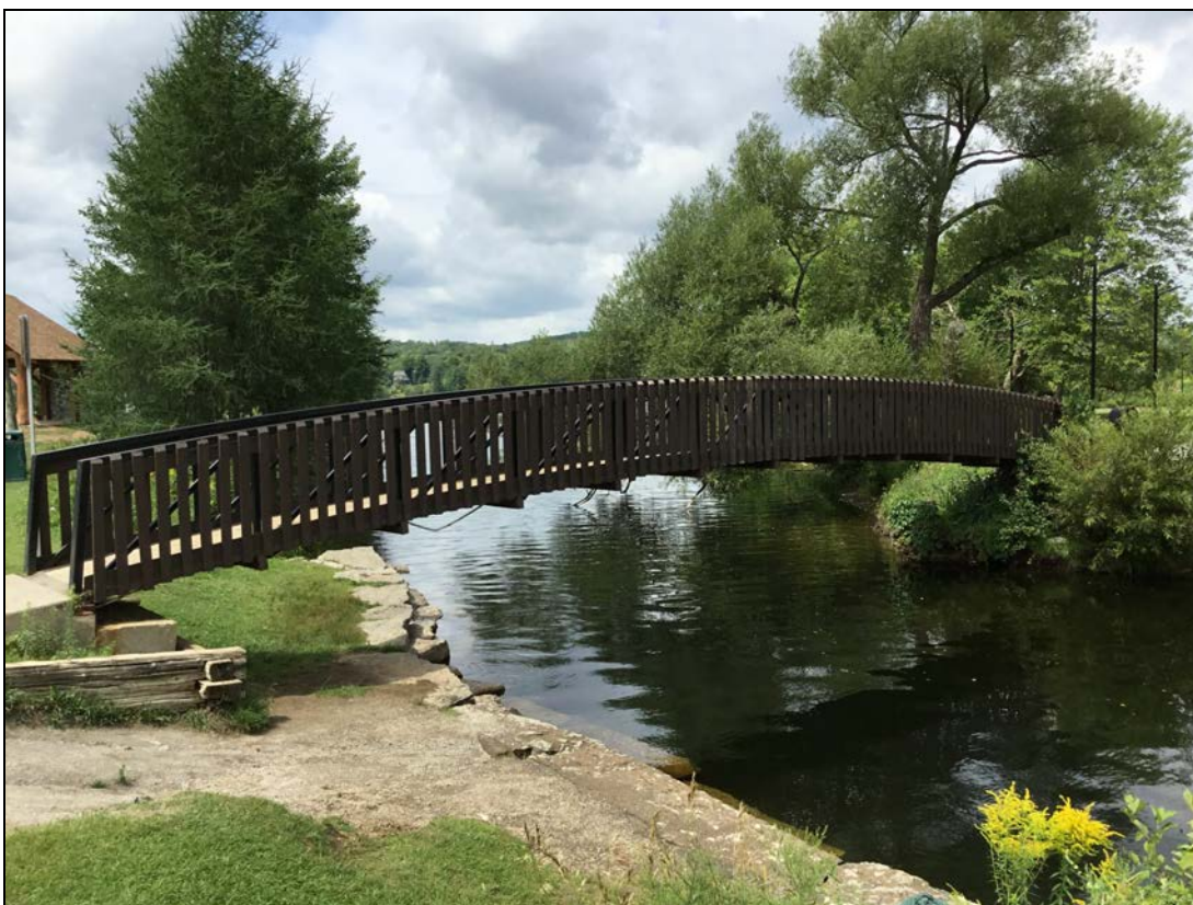
Description: General elevation, east.
