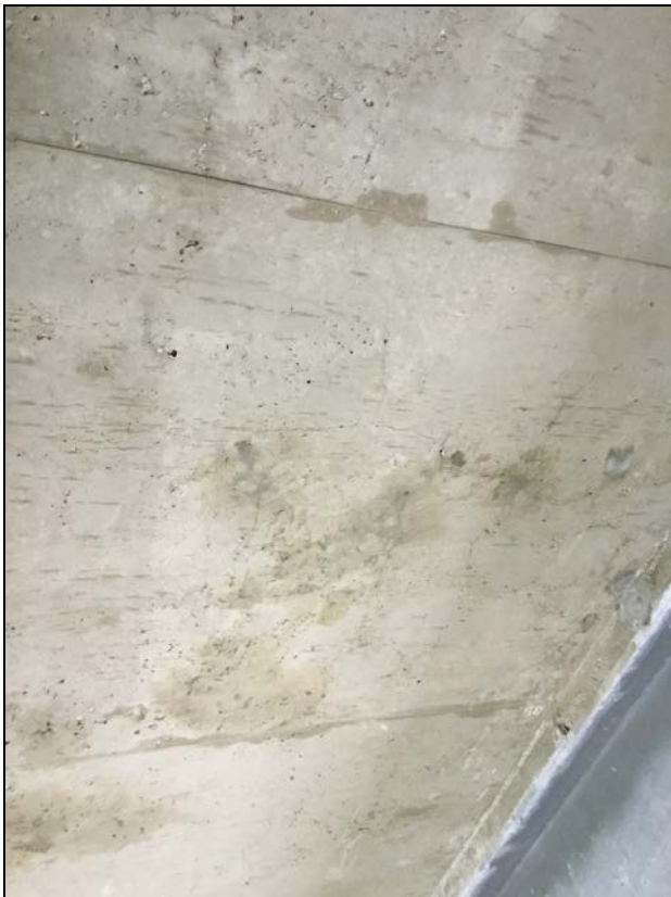
Decks / Soffit - Thin Slab
