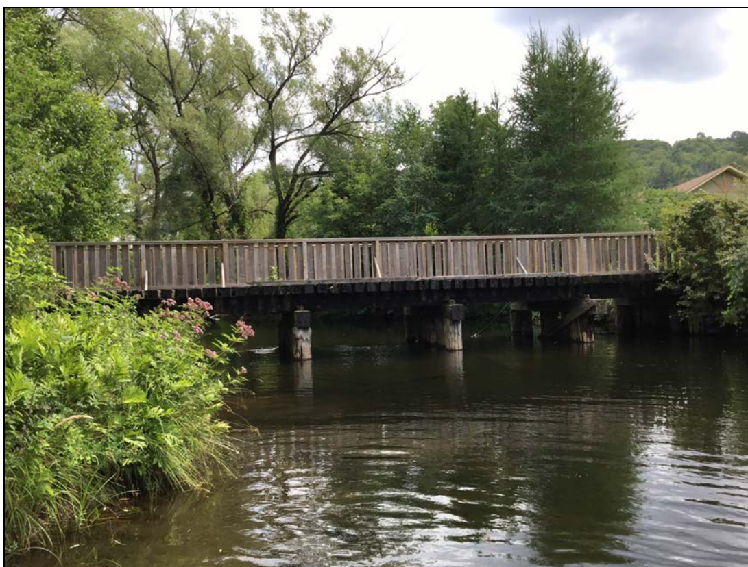
Description: General elevation, west.
