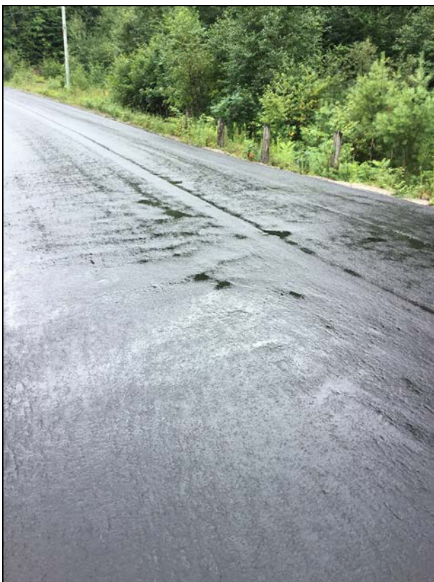
Description: General condition, some minor rippling. Decks / Wearing Surface (Top)
