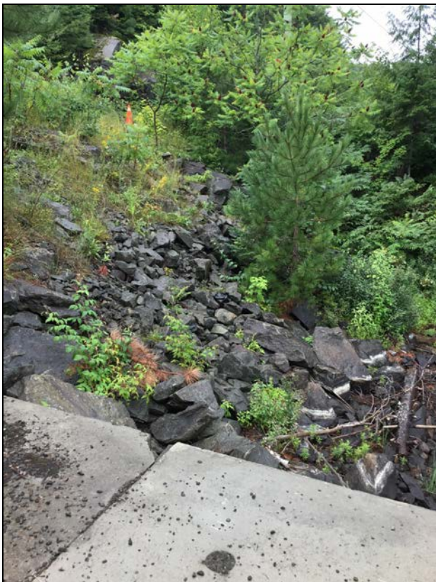
Description: Northeast embankment.
