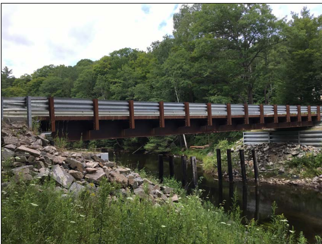
Description: East elevation
