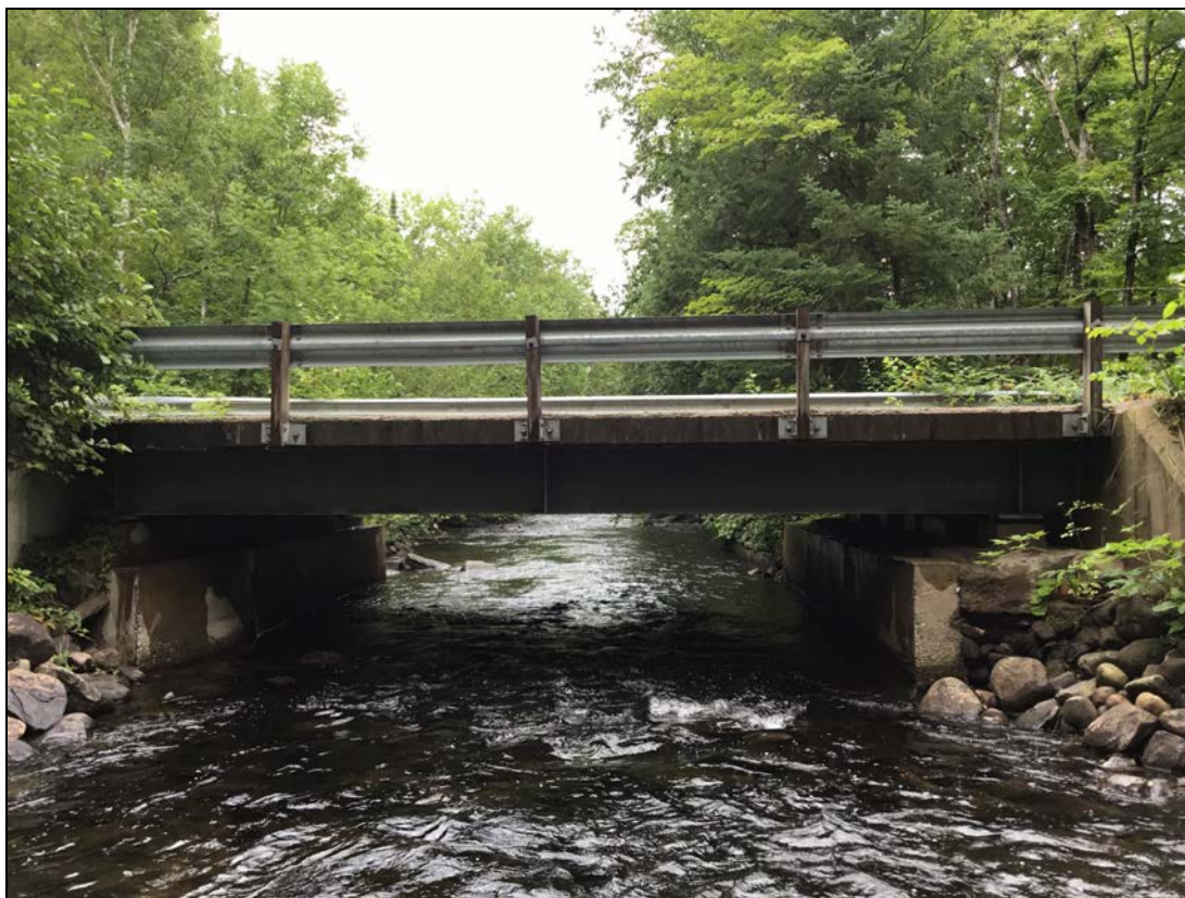
Description: General elevation, west.
