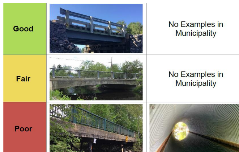
Figure 18 Bridges and Culverts Condition Images
