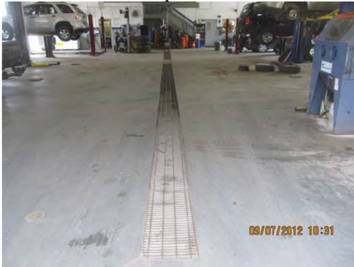
Oil water separator access cover in shop
