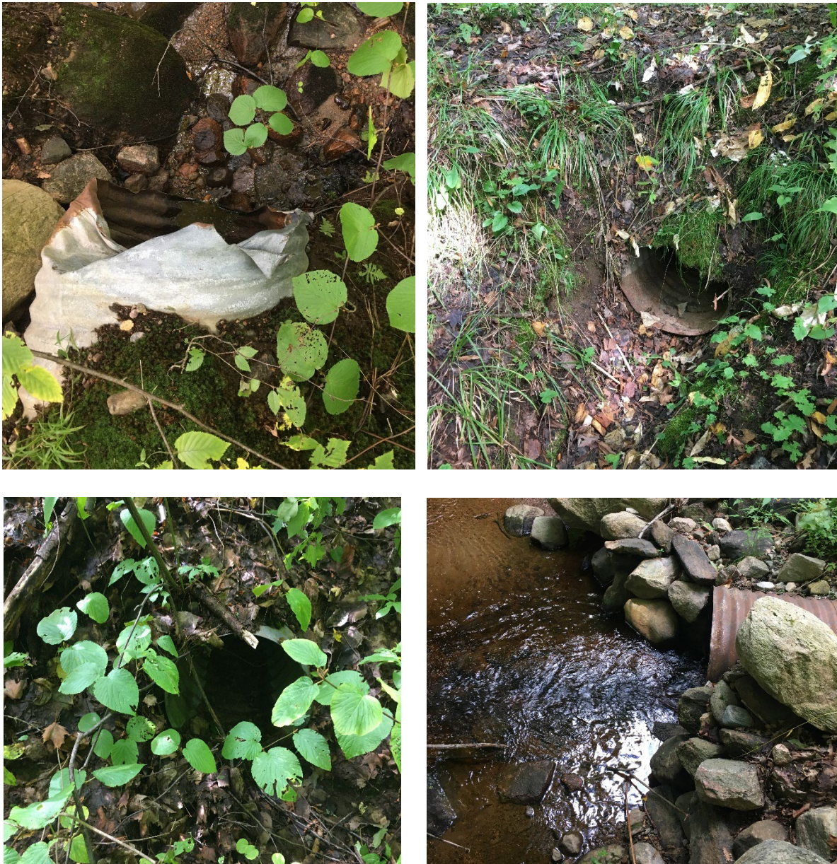
Figure 7- Existing CSP culverts
